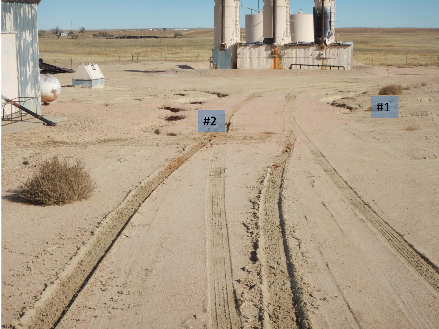
Photo 2: Photo taken from southwestern end of location, facing east. Note the erosion in center-right and center-left of photo forming stormwater erosion channels #1 and #2.
