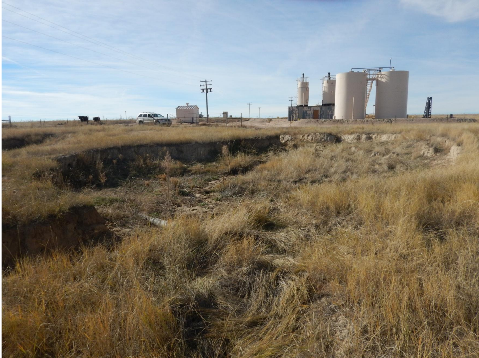
Photo 19: Photo taken east of location facing west towards location. Photo of “washed out”, eroded area.
