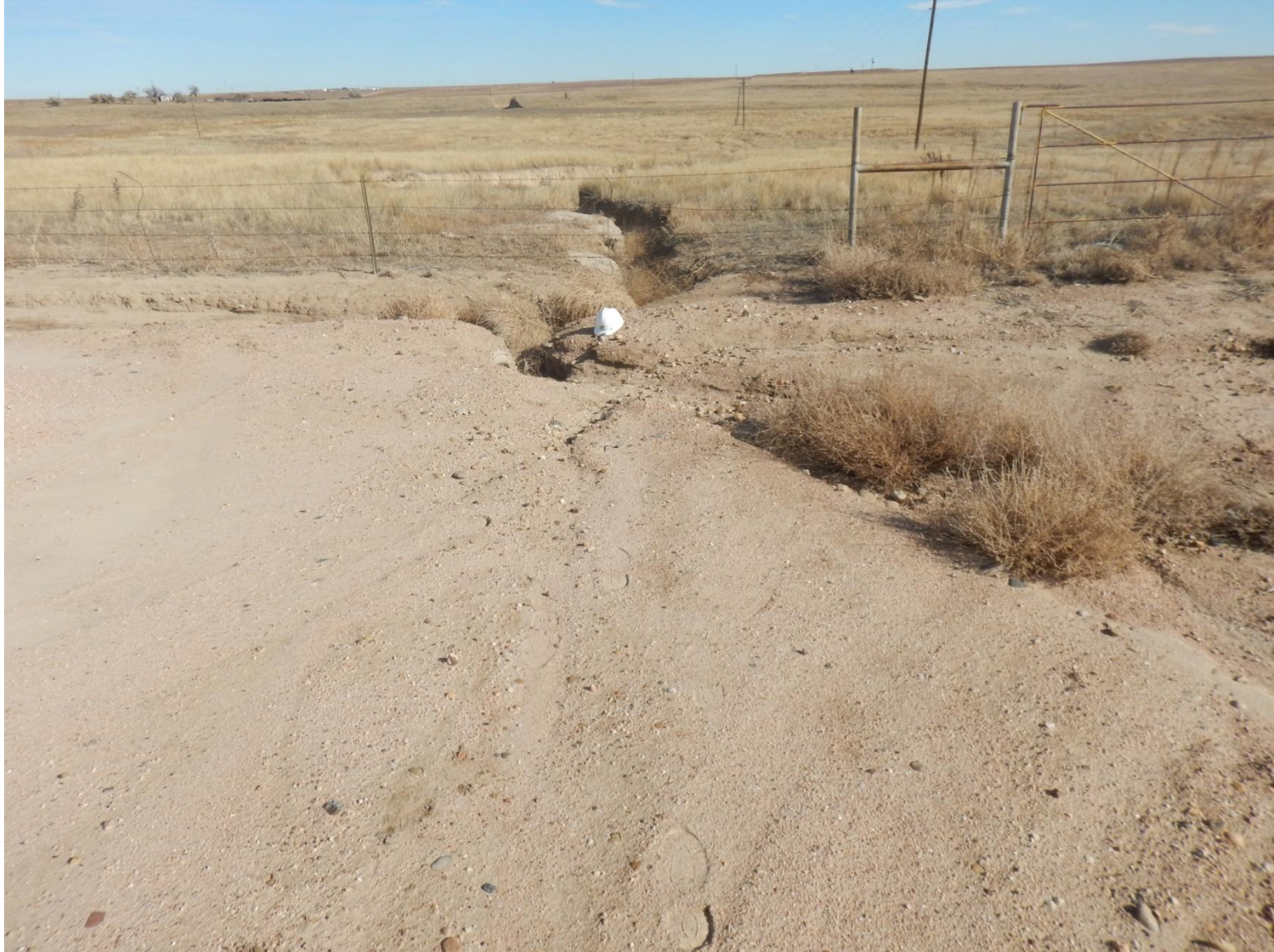
Photo 15: Photo taken from east end of location, facing east. Photo shows confluence of storm water erosion channels from northern and southern halves of location, leading off location
