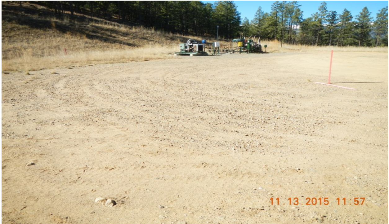
photo 4: Facing west towards the production equipment.
