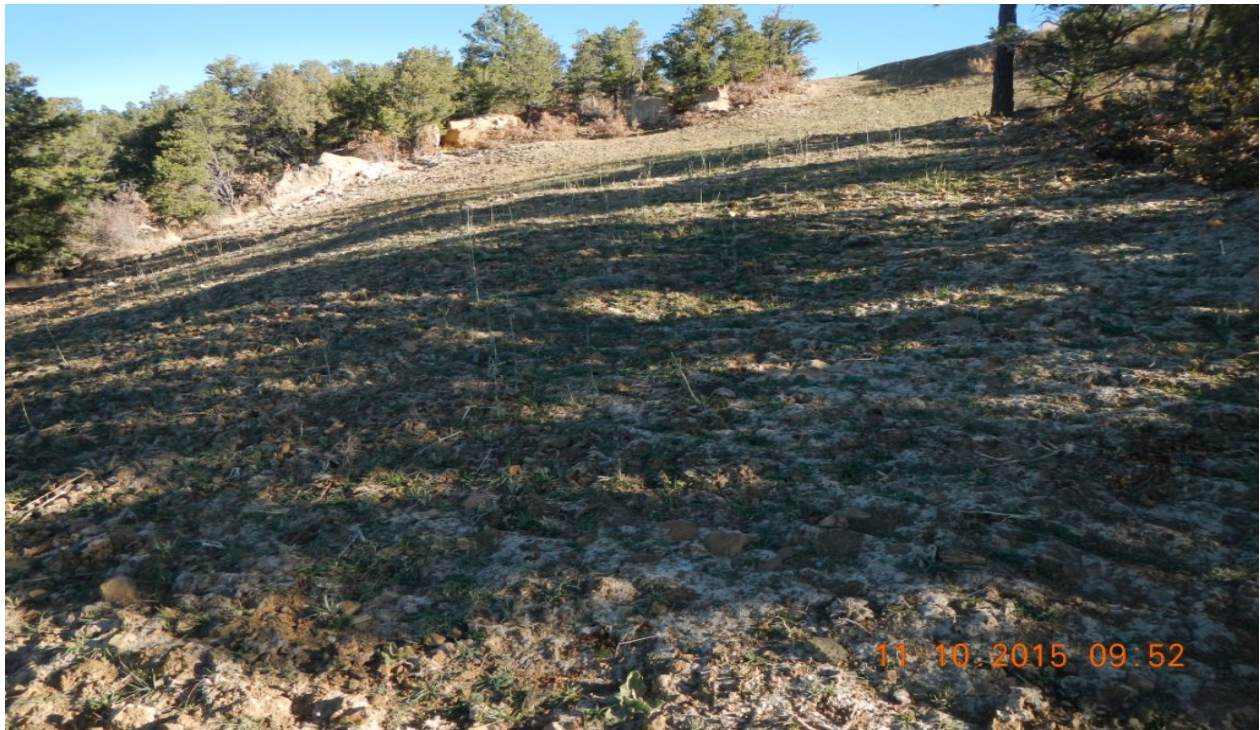
photo 7: Facing north along the reclaimed access road.
