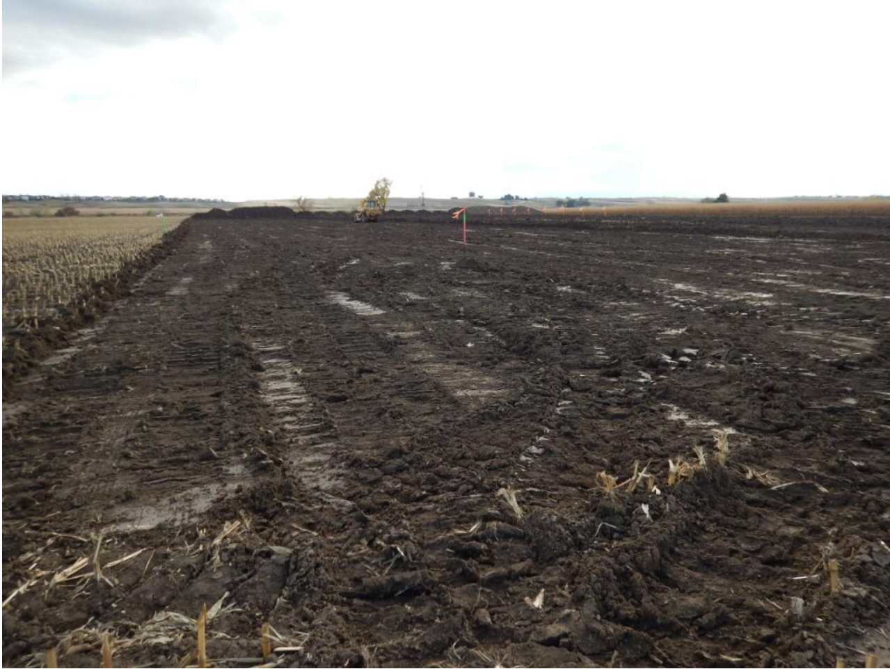
Photo 7. Photo taken of northern location, facing South. Topsoil removal in process.
