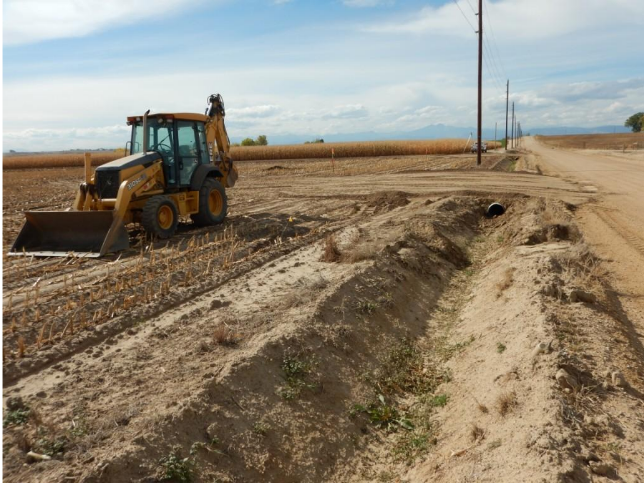
Photo 1. Photo taken of east, northern access road, facing West. Stormwater control ditch with culvert in center of photo.
