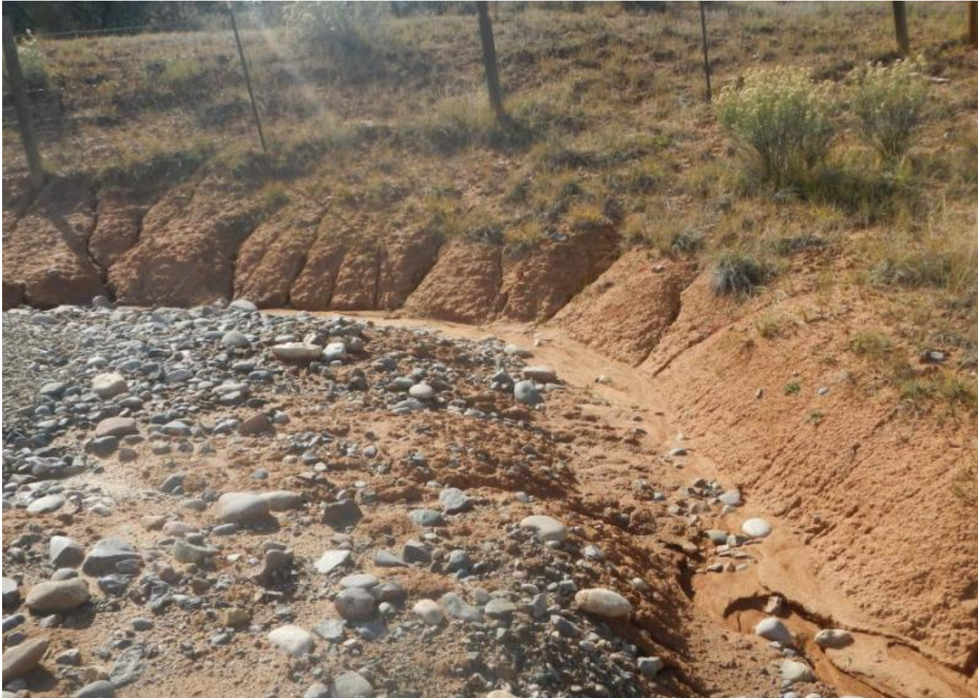
Photo 2. View of area where significant erosion begins within stormwater diversion in northwestern corner of working area.
