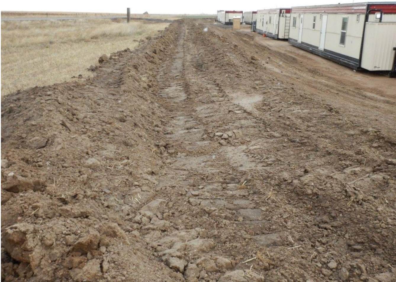
Photo 7. Photo taken from northwest location, facing East. Stormwater control ditch installed in center of photo.
