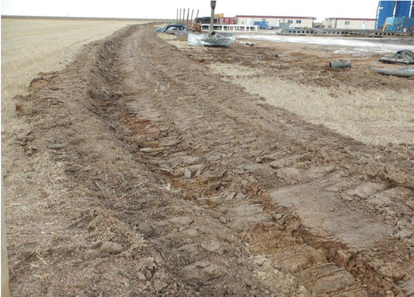
Photo 5. Photo taken from southwest location, facing North. Stormwater control ditch installed in center of photo.
