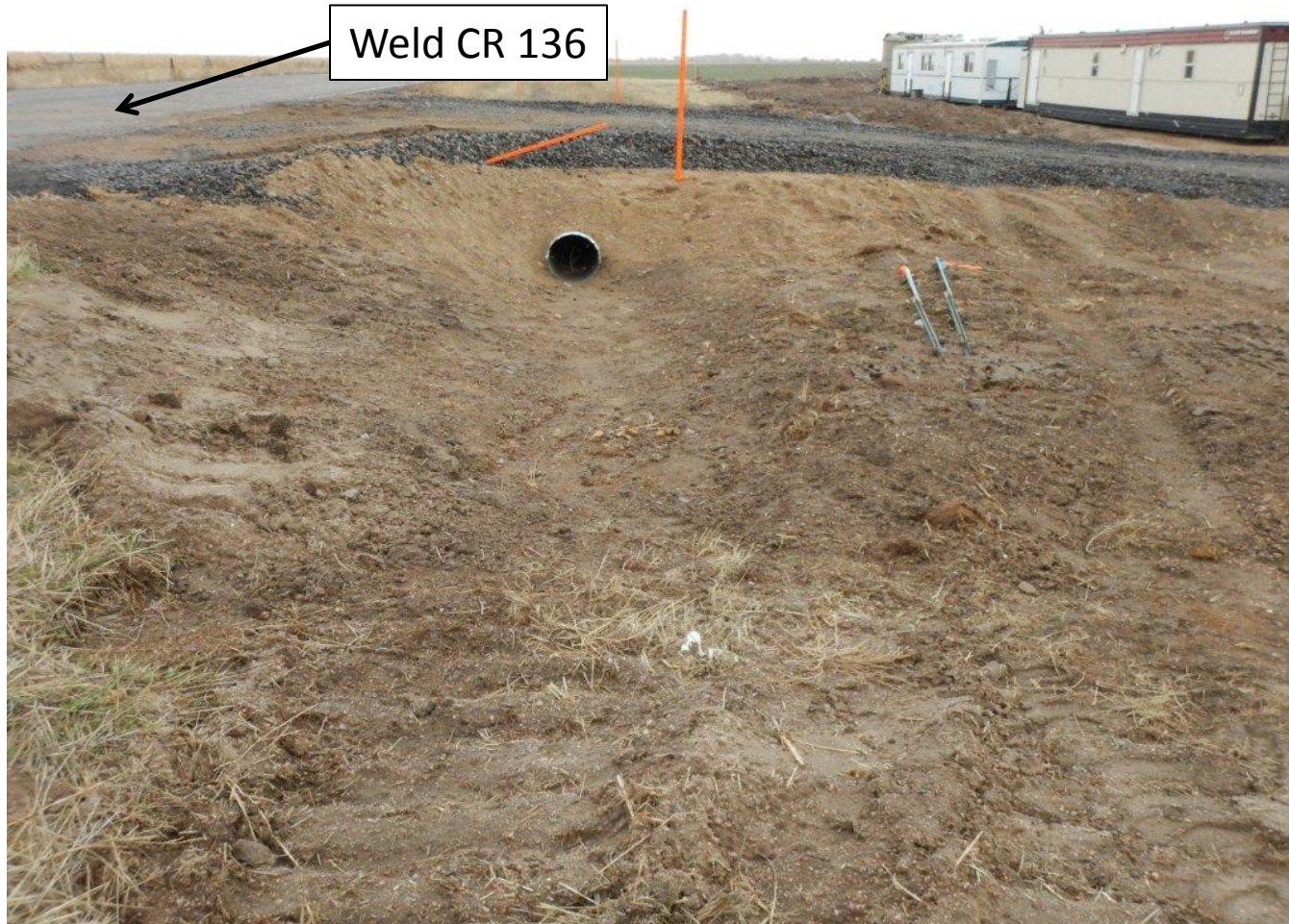
Photo 1. Photo taken from north access road with stormwater BMP's installed, facing East.
