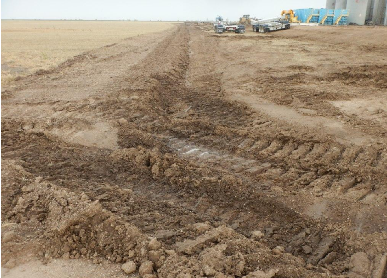
Photo 4. Photo taken from southeast location, facing West. Stormwater control ditch installed in center of photo.
