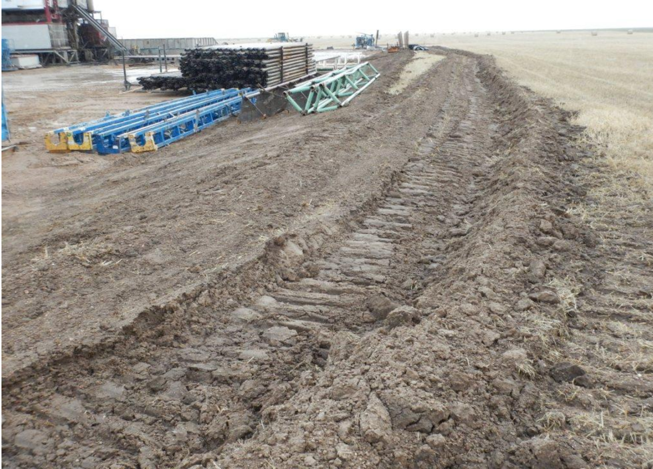
Photo 6. Photo taken from northwest location, facing South. Stormwater control ditch installed in center of photo.
