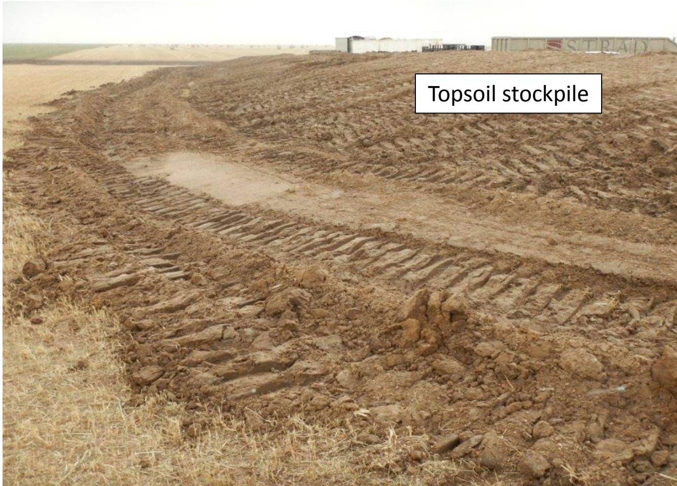
Photo 3. Photo taken from east topsoil stockpile location, facing South. Stormwater control ditch installed in center of photo and stabilized topsoil stockpile.
