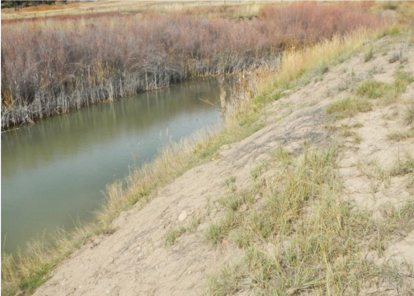
Photo 4. View of open water adjacent to northern portion of the project area. Vegetation on slope appears to be sufficiently stabilizing the slope at this time.
