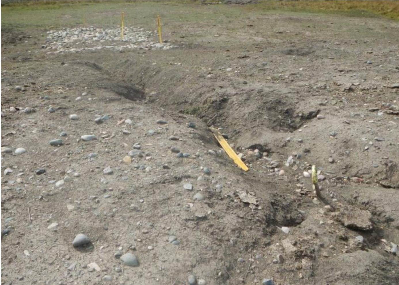
Photo 2. View of erosional channel (approximately 2 feet wide and 1 foot deep) and damaged anchor marker in southwestern portion of project area.
