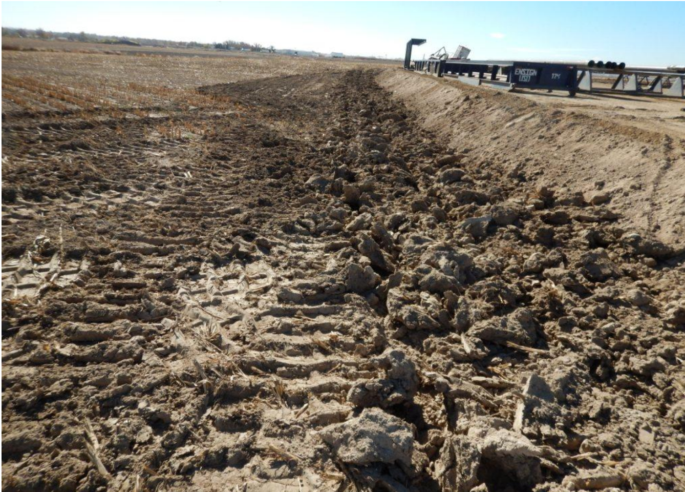
Photo 2. Photo taken from southeast location, facing Southwest. Need to install stormwater control ditch. Surface roughening is inadequate.
