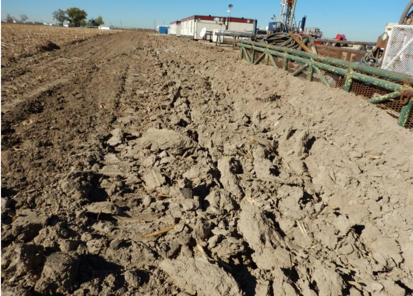
Photo 3. Photo taken from western location, facing Northwest. Need to install stormwater control ditch. Surface roughening is inadequate.
