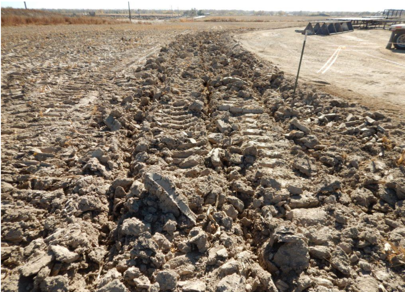
Photo 1. Photo taken from southeast location, facing South. Need to install stormwater control ditch. Surface roughening is inadequate.
