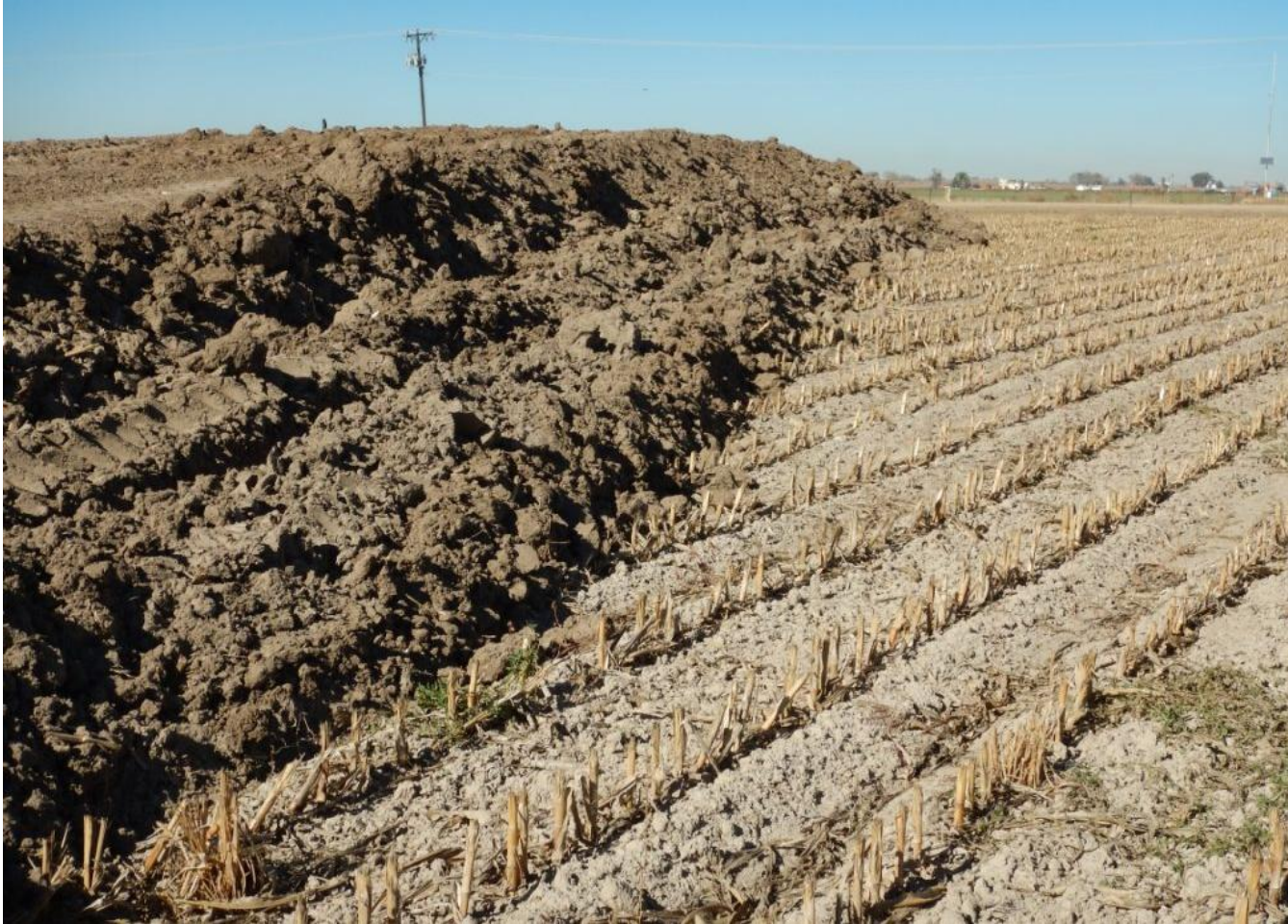
Photo 4. Photo taken from eastern topsoil location, facing North. Need to install stormwater control ditch around topsoil stockpile to prevent the loss of topsoil offsite.
