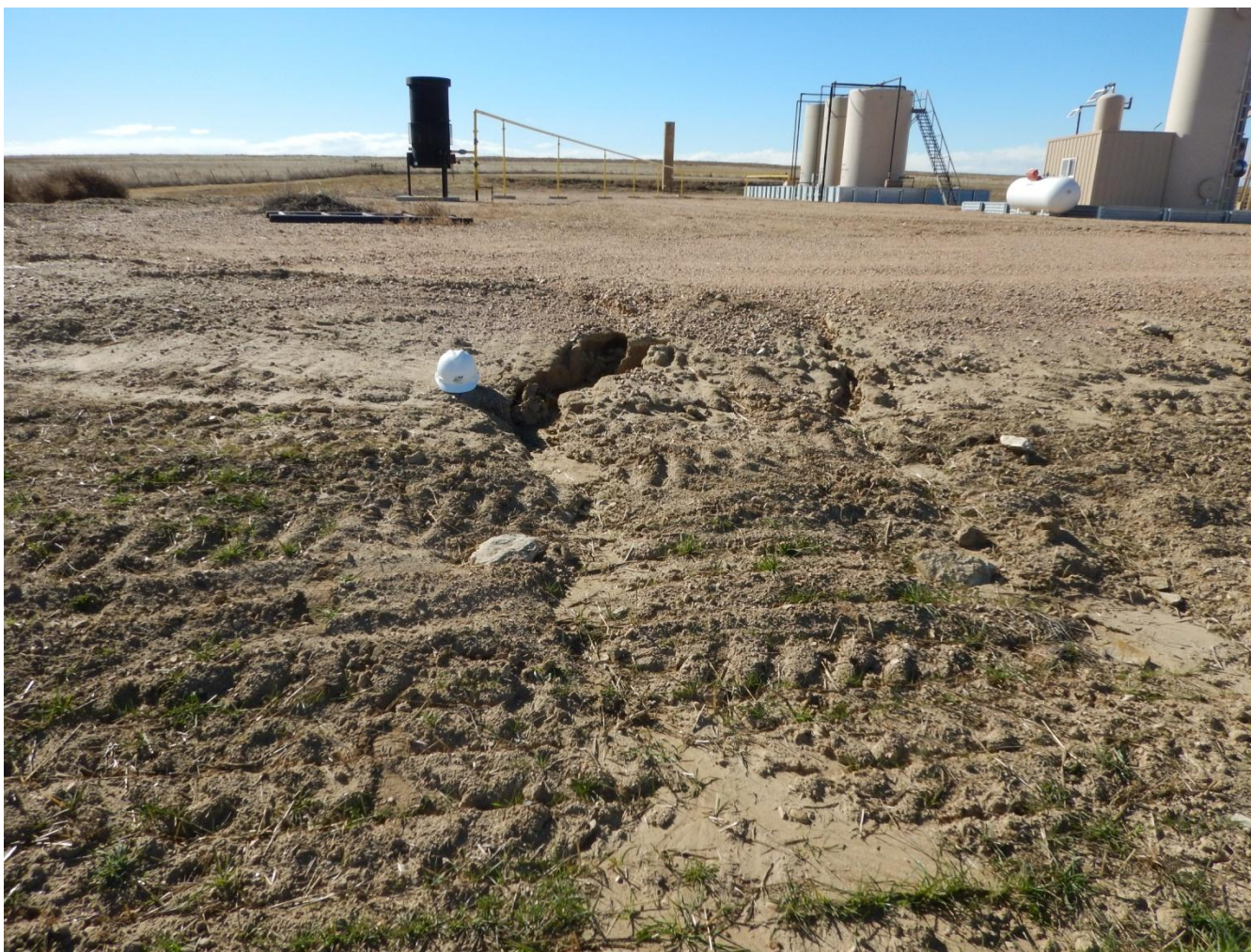
Photo 6: Photo from Southeast portion of location. Photo of rill erosion on slope.
