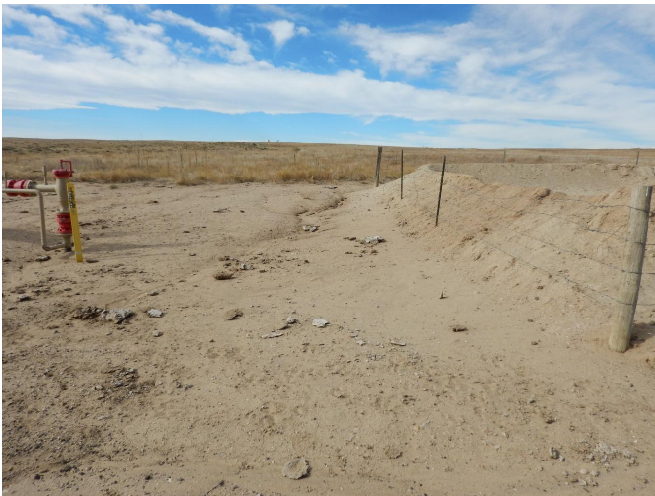
Photo 7: Photo taken from battery location facing west. Note the rill erosion developing on site.
