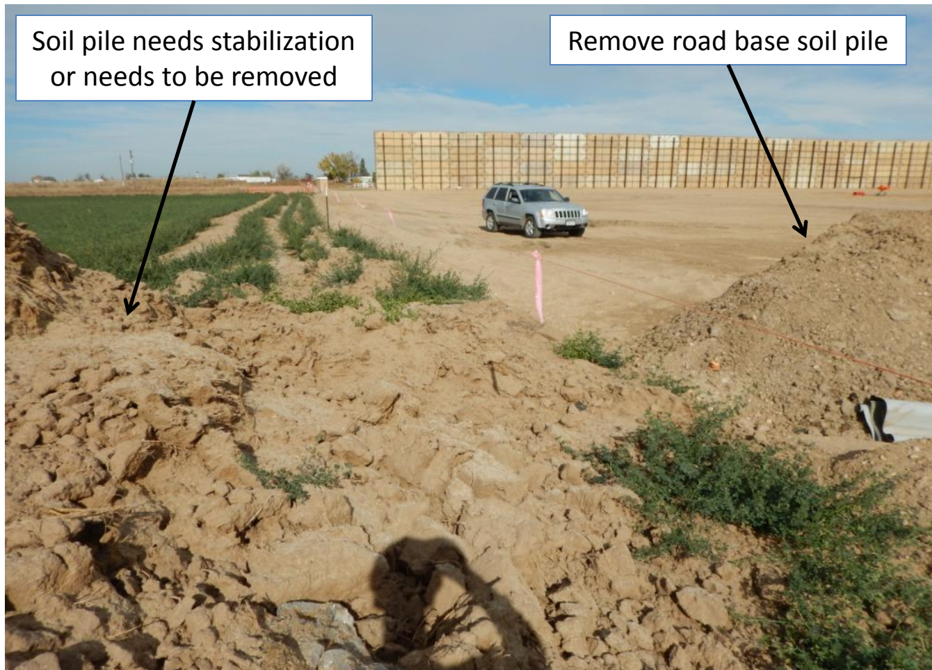
Photo 3. Photo taken from southwest location, facing North. Need to stabilize soil pile from sediment erosion or needs to be removed, and remove road base soil pile.
