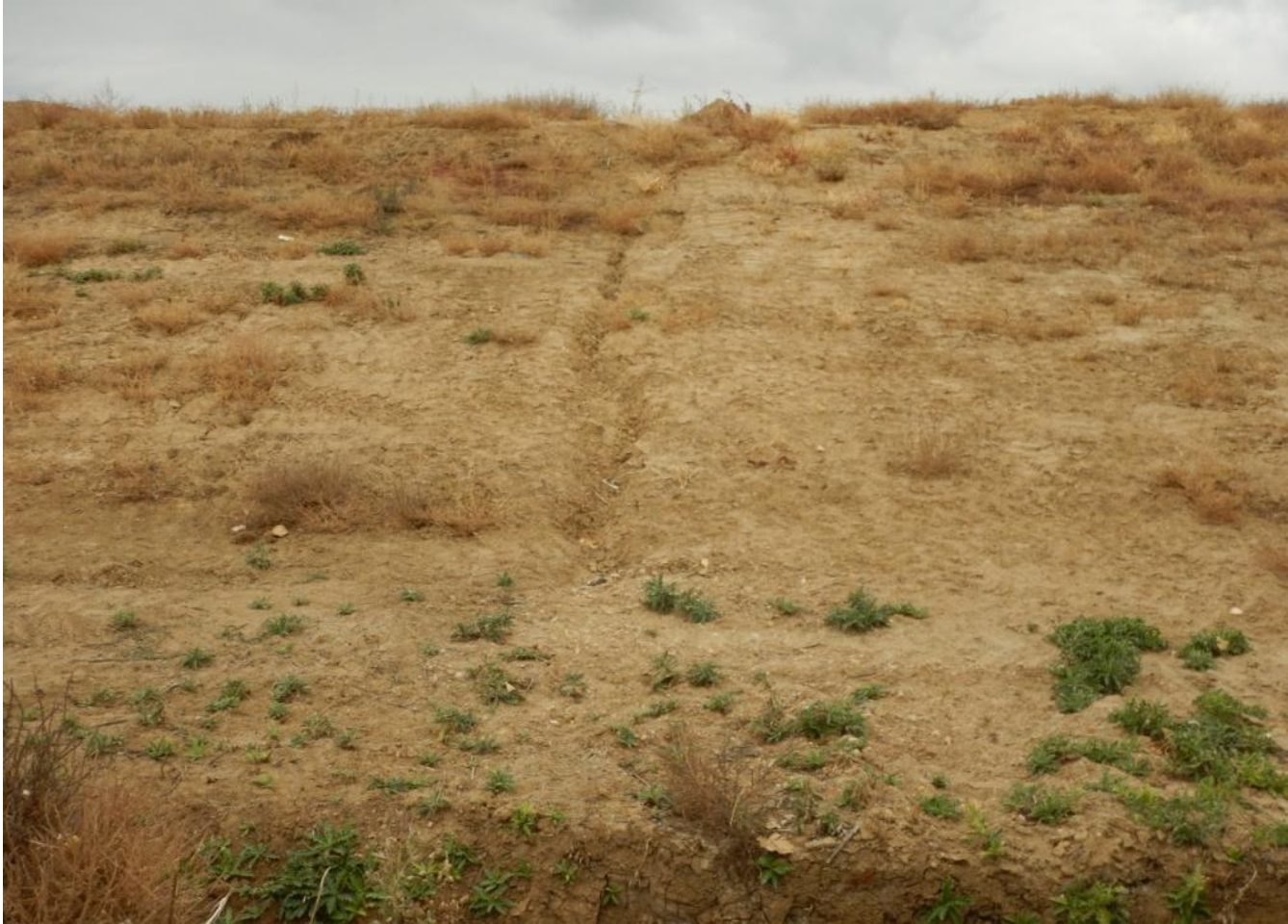
Photo 22. Photo taken from east location, facing West. Sediment movement and erosion needs to be controlled. Weed maintenance is needed.
