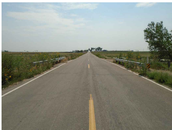
VIEW SOUTH (COUNTY ROAD 59)
