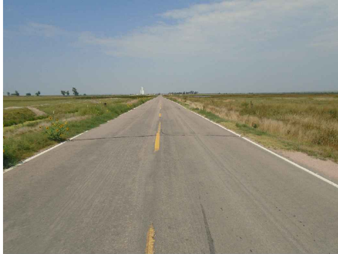
VIEW NORTH (COUNTY ROAD 59)
