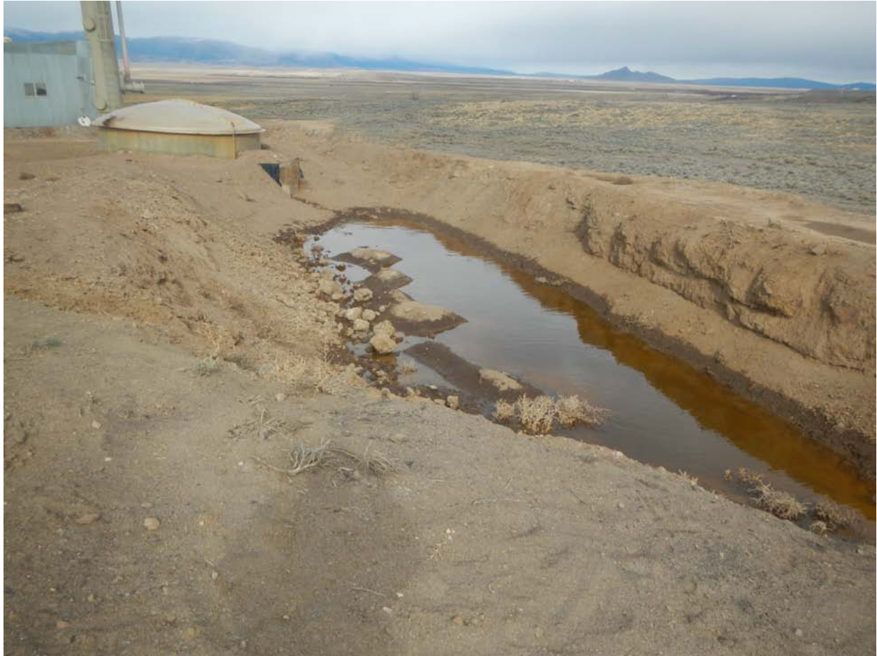
Pit facility 111692, water observed in pit, recent weather was rainy/snowy. Water has odor. Indication that water came from production observable in wet soil from valve box.
