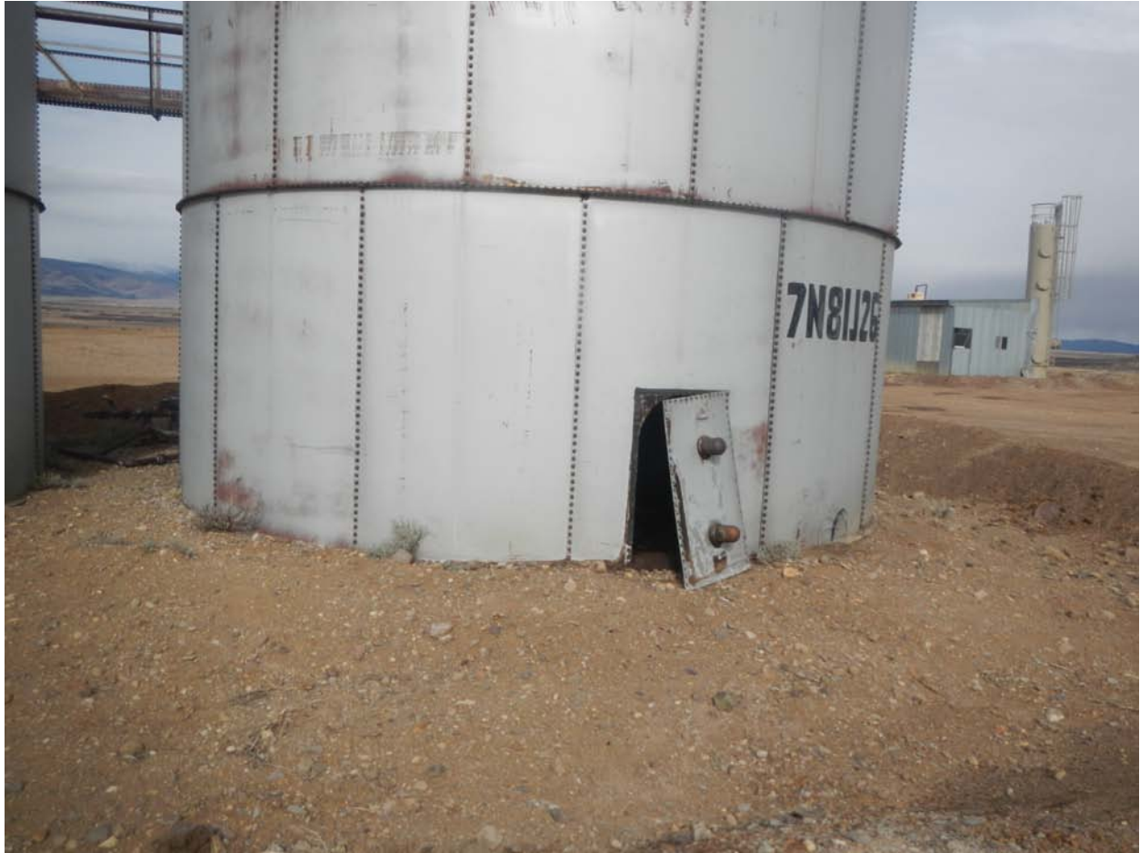
500 bbl tank, access panel open, no fluid observed leaving tank.
