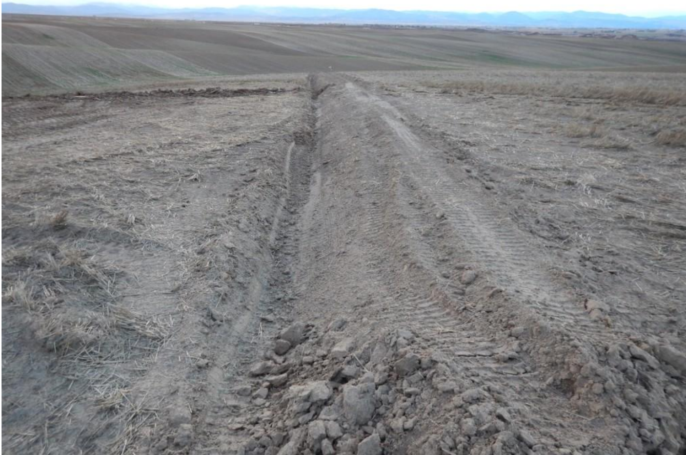
Photo 12. Photo taken from southwest location of facility pad, facing West. Stormwater control ditch located in center of photo heading West from sediment catch.
