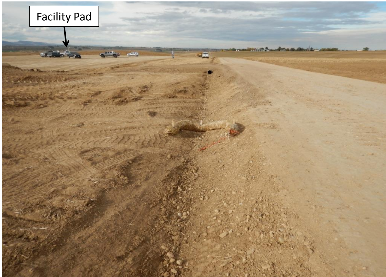
Photo 17. Photo taken from eastern edge of facility pad and well pad, facing North. Stormwater control ditch, culvert, and straw wattle in center of photo for access road.
