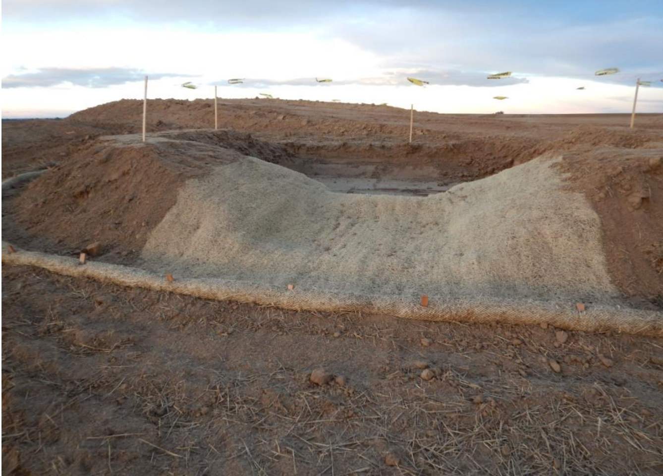
Photo 11. Photo taken from southwest location of facility pad, facing Northeast. Stormwater sediment catch located in center of photo.
