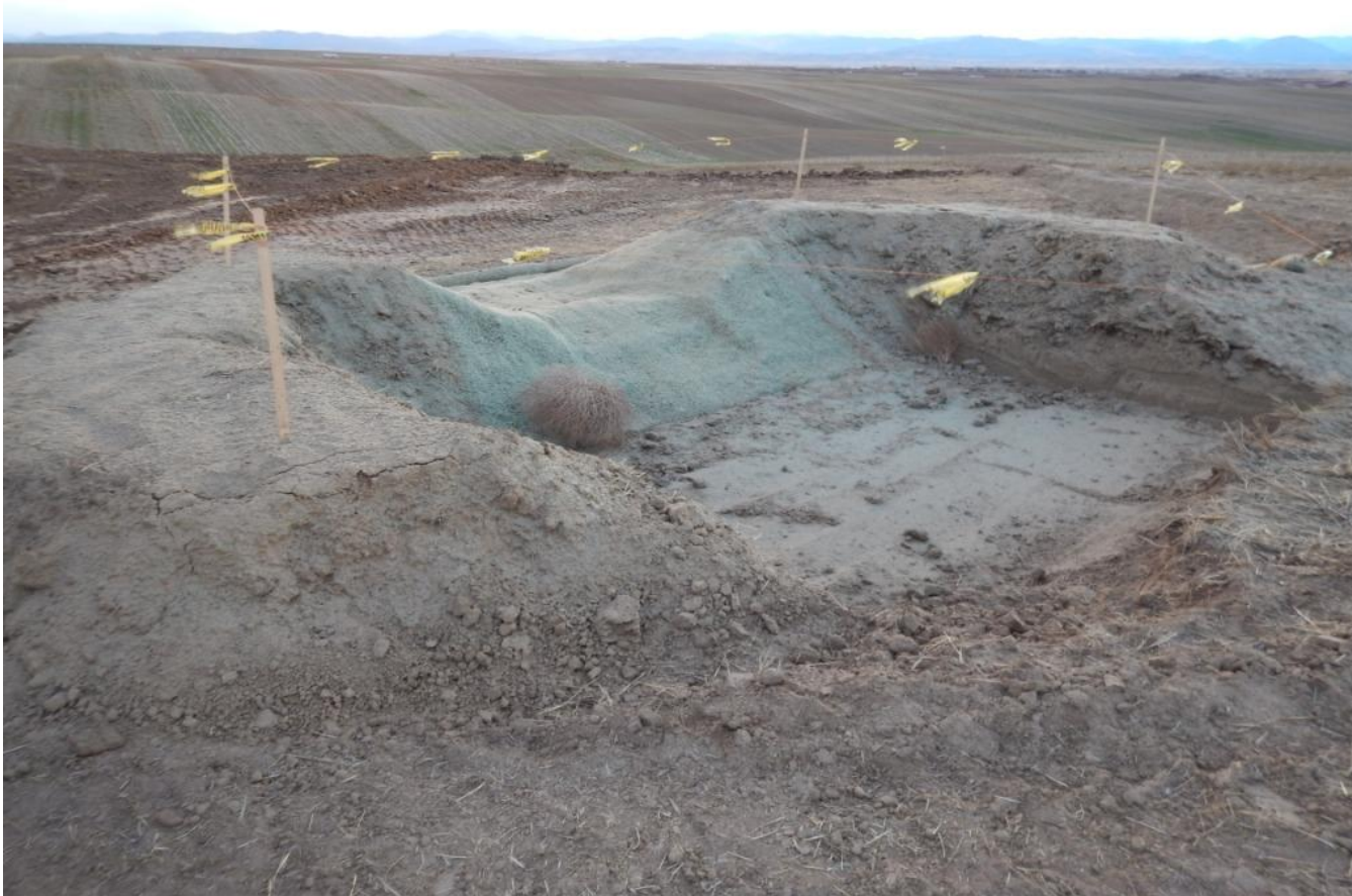
Photo 10. Photo taken from southwest location of facility pad, facing West. Stormwater sediment catch located in center of photo.
