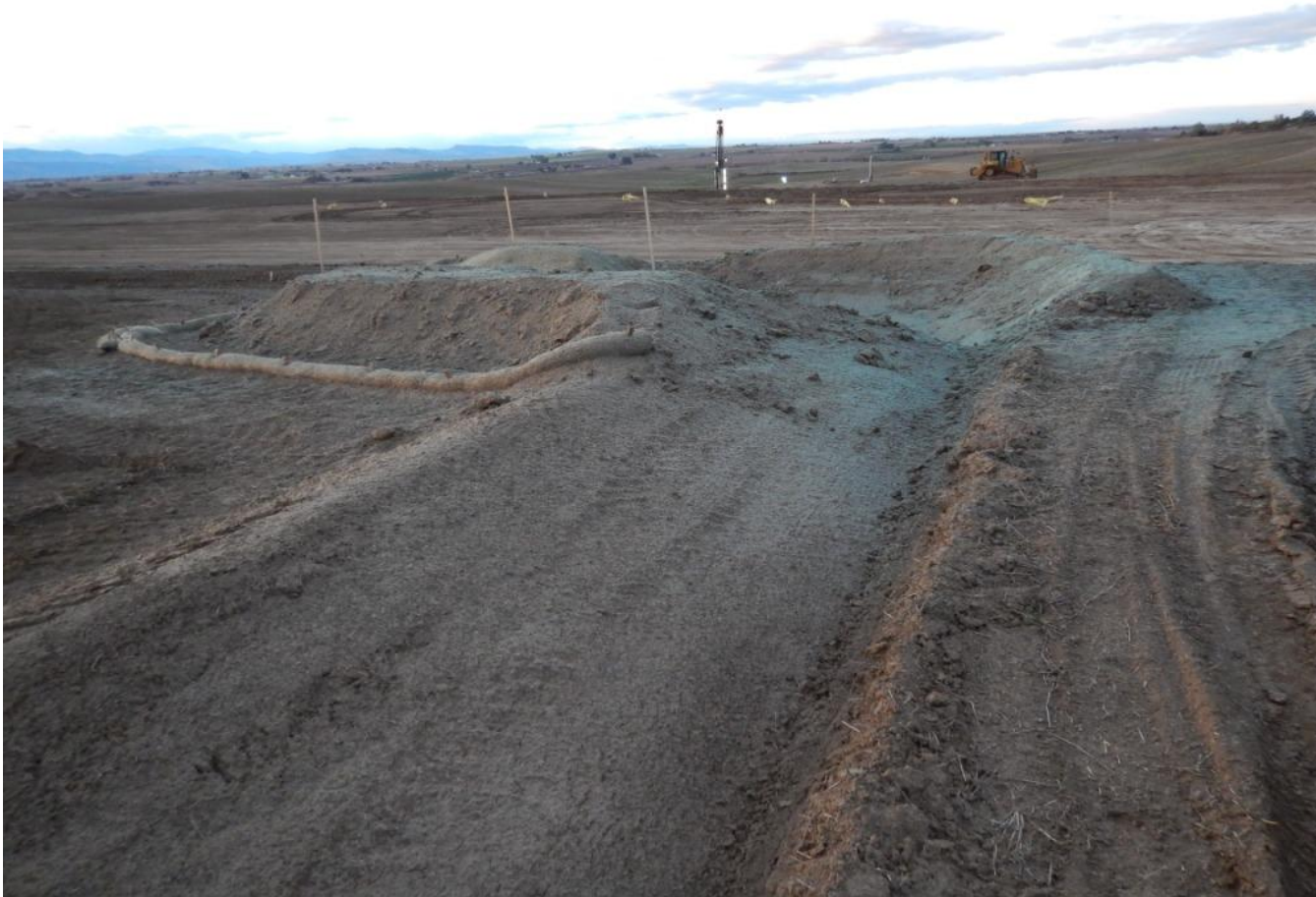
Photo 14. Photo taken from northwest location of facility pad, facing North. Stormwater sediment catch located in center of photo.
