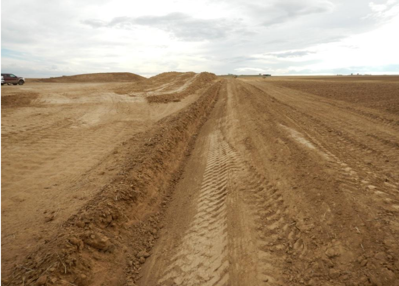
Photo 9. Photo taken from western edge of facility pad, facing south. Stormwater control ditch located in center of photo.
