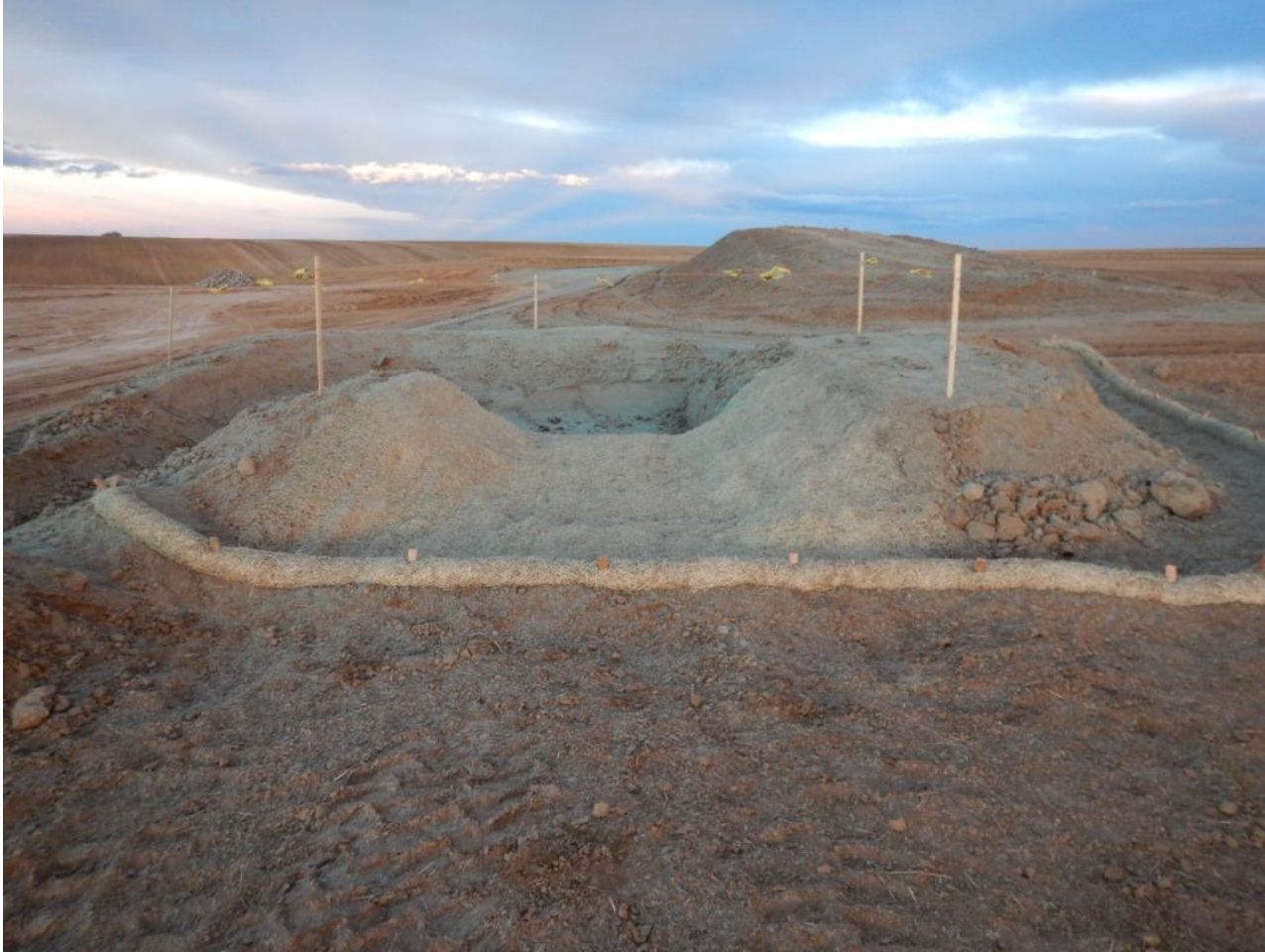
Photo 15. Photo taken from northwest location of facility pad, facing East towards north topsoil stockpile. Stormwater sediment catch located in center of photo.
