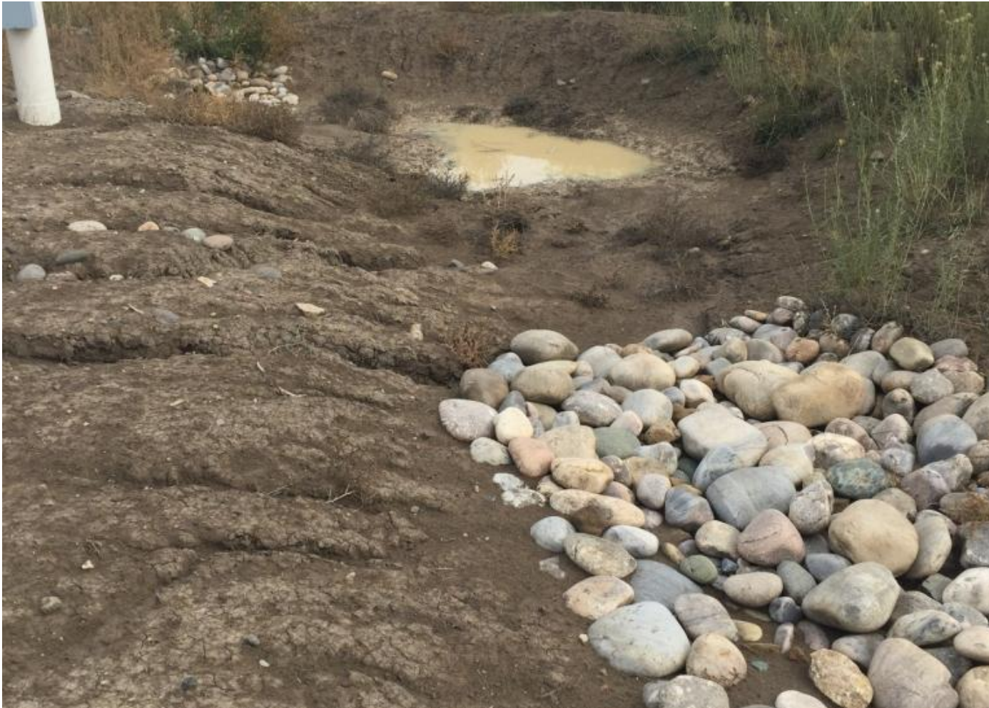
Photo 2. View of stormwater BMP (cobble lining and silt trap) within northeastern portion of the project area.
