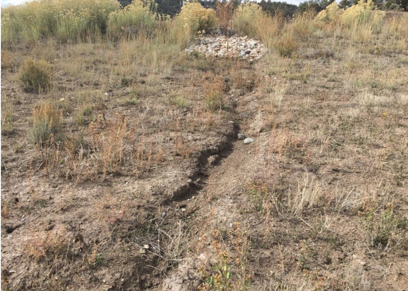
Photo 3. View of erosional channel (approximately 1.5 feet wide and 8 inches deep) forming downstream of stormwater BMP in northeastern portion of the project area.
