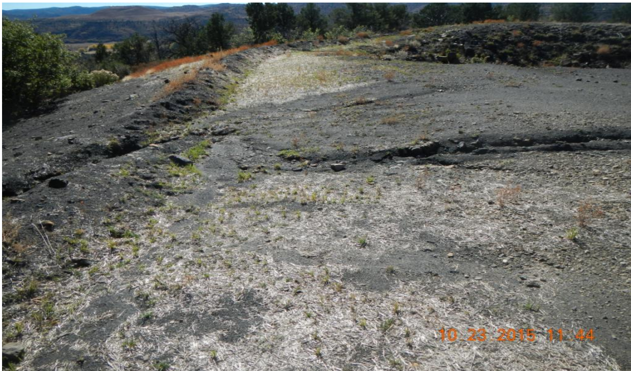
photo 4: East side of the location facing south. Erosion channel developing on the pad.
