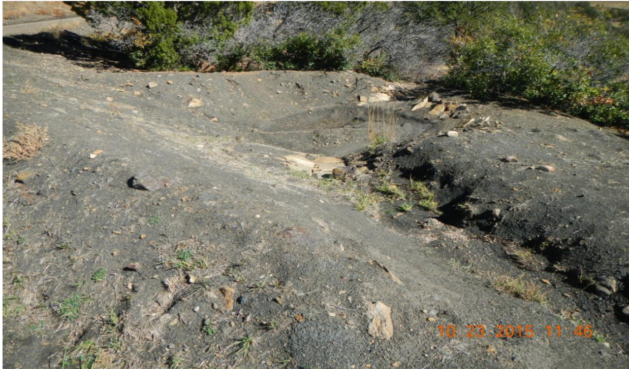
photo 5: Sediment trap at the northeast corner of location is filling up with sediment.
