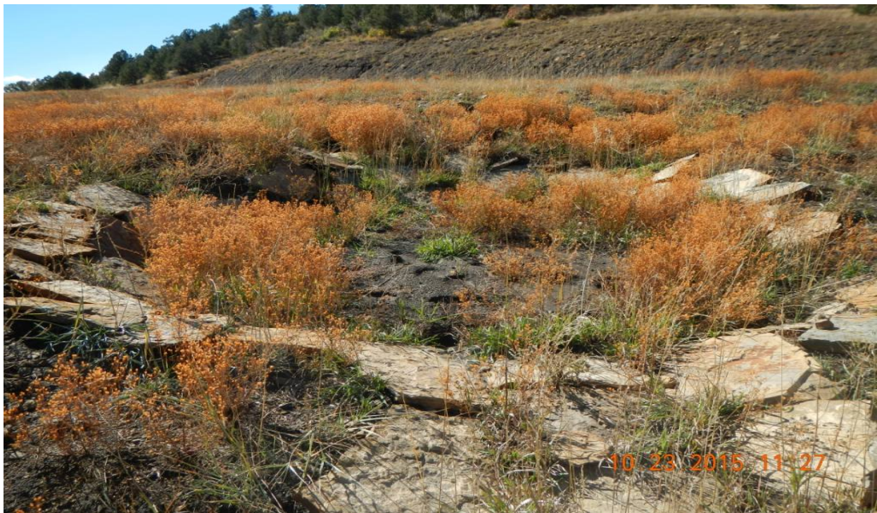
photo 16: Northeast corner of the location facing southwest. Sediment trap is filled with sediment.
