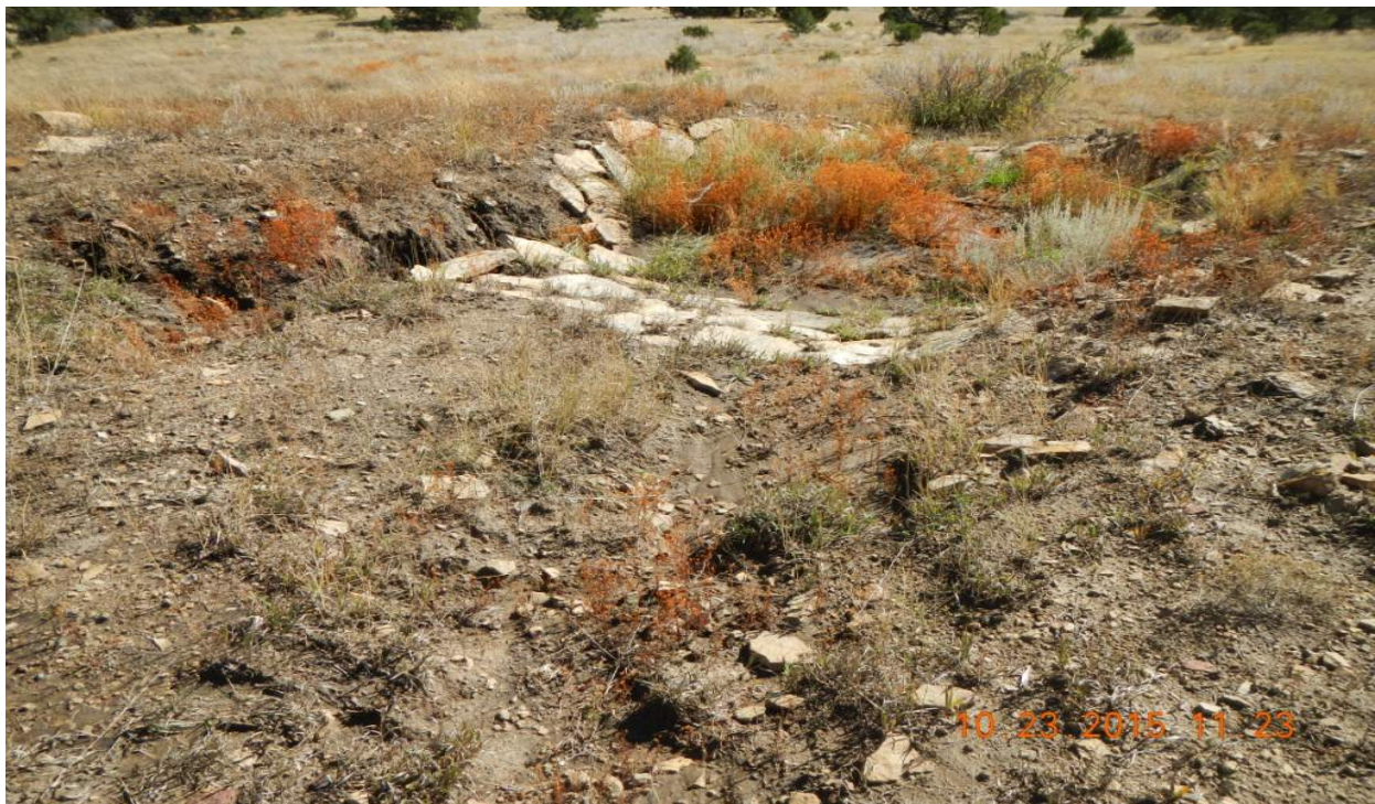
photo 14: Sediment trap the the southeast corner of location is filled with sediment.
