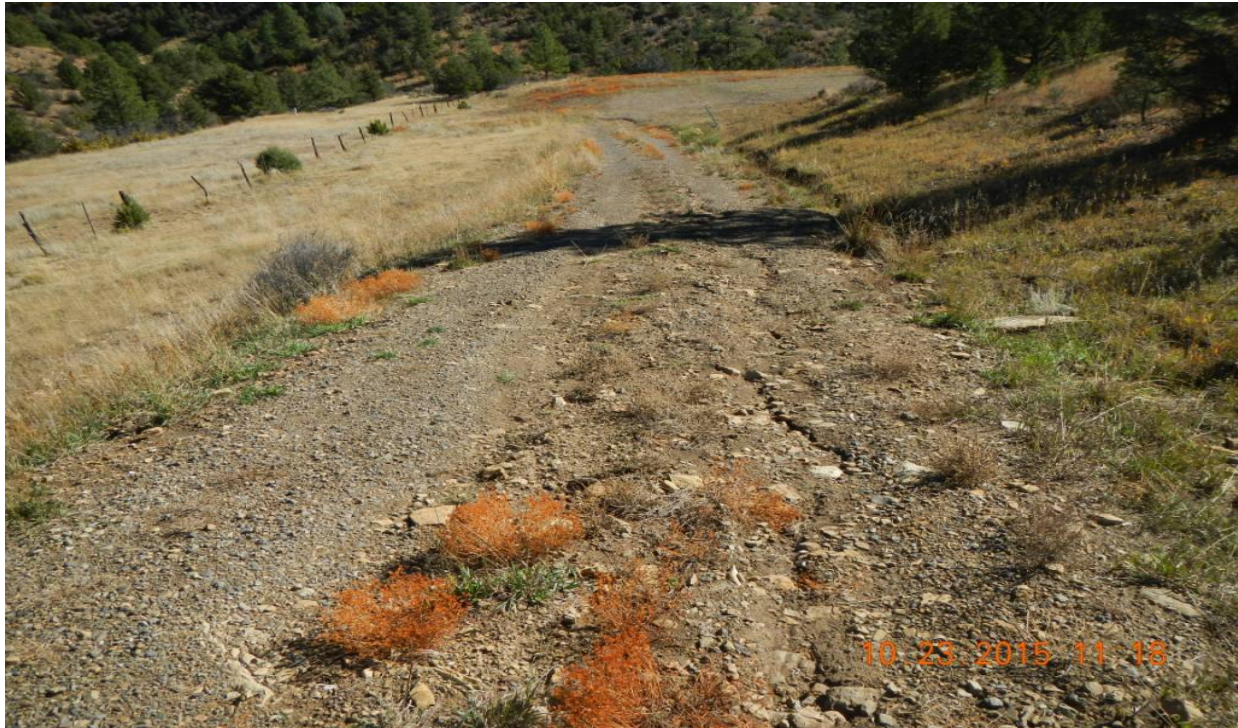
photo 7: Facing east towards the location.
