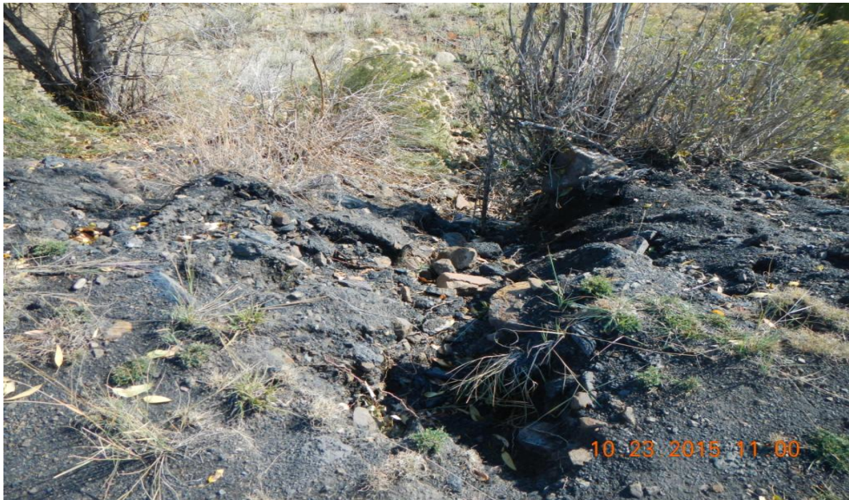
photo 5: Erosional channel has developed off the east side of the pad.
