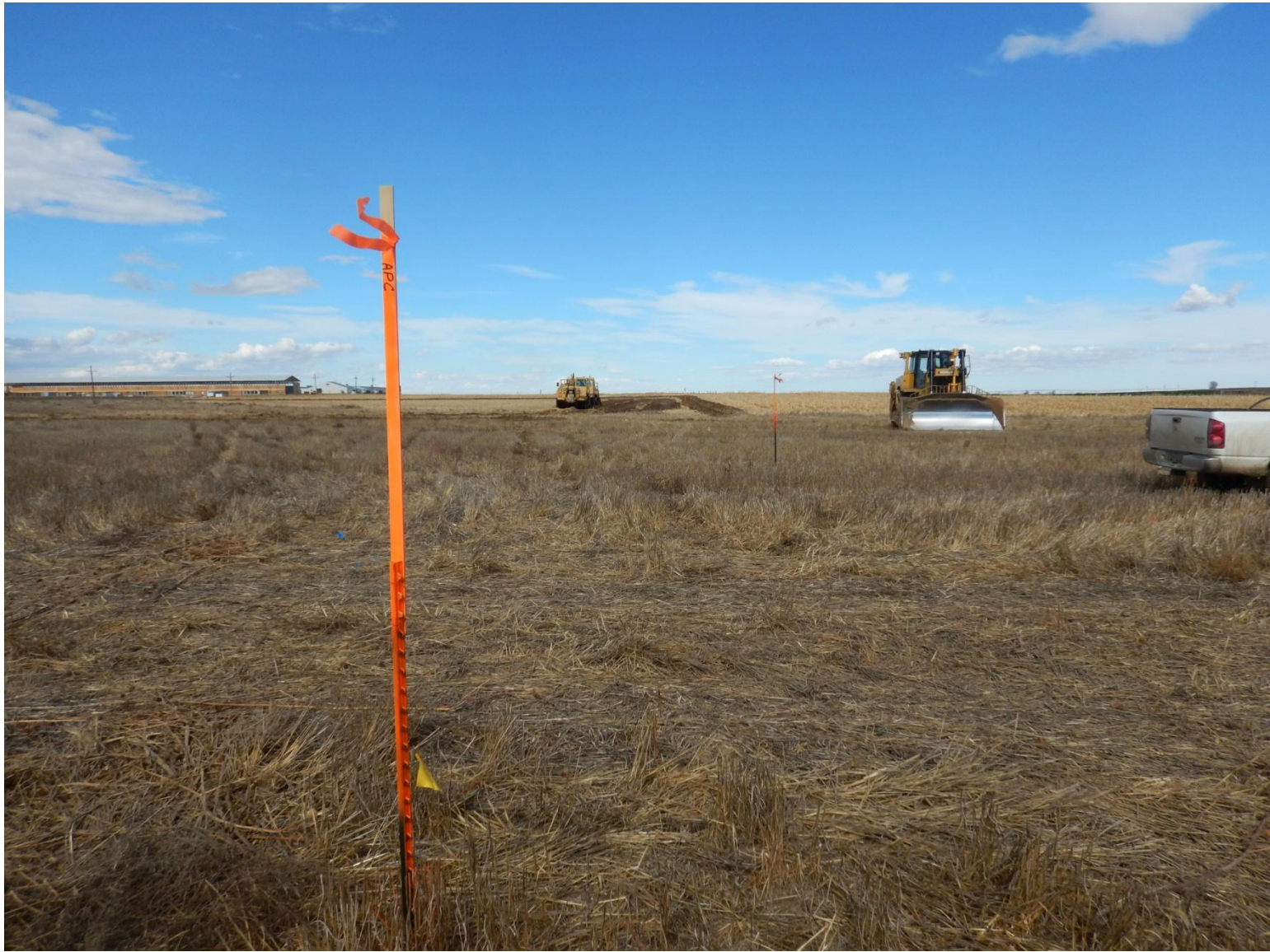
Photo 1: Photo taken from South side of location looking North.
