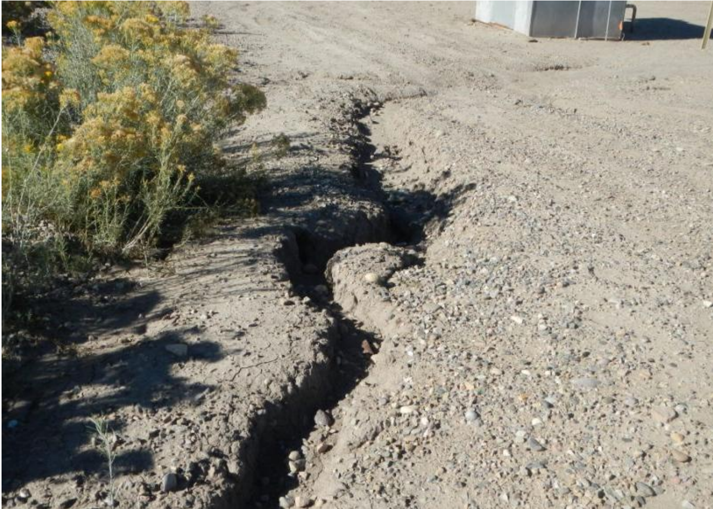
Photo 2. View of erosional channel at well pad entrance flowing across well pad toward the northern edge. Channel is approximately 1.5 feet wide and deep.
