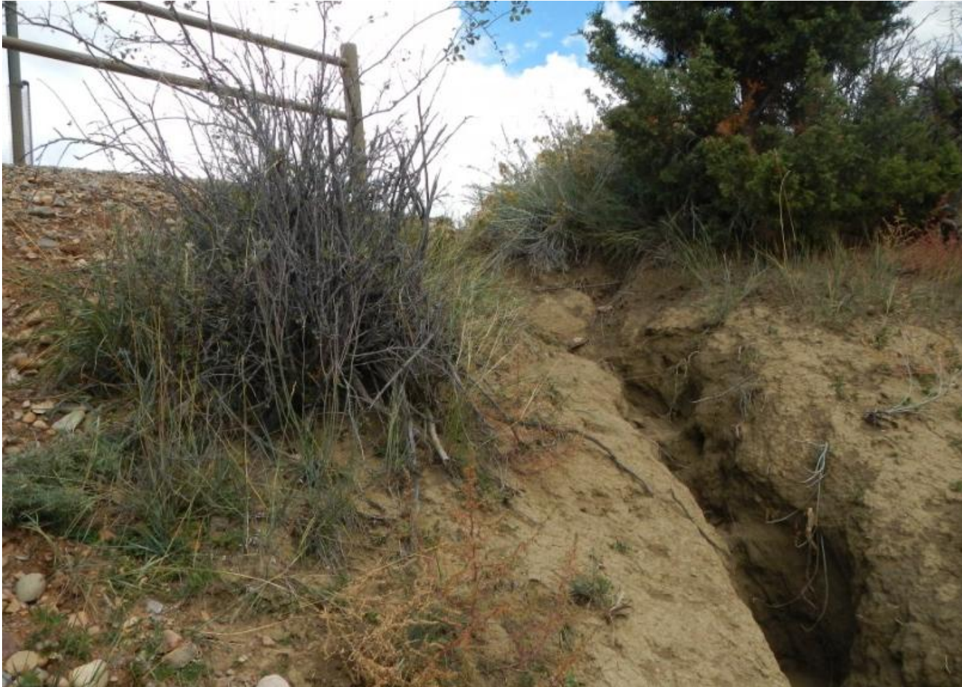
Photo 4. View of erosional channel eroding the southern edge of working area on the portion of the well pad that is west and elevated from the eastern portion (Facing upslope). This erosional channel is approximately 2 feet wide and up to 4 feet deep and eroding directly into the Florida River.
