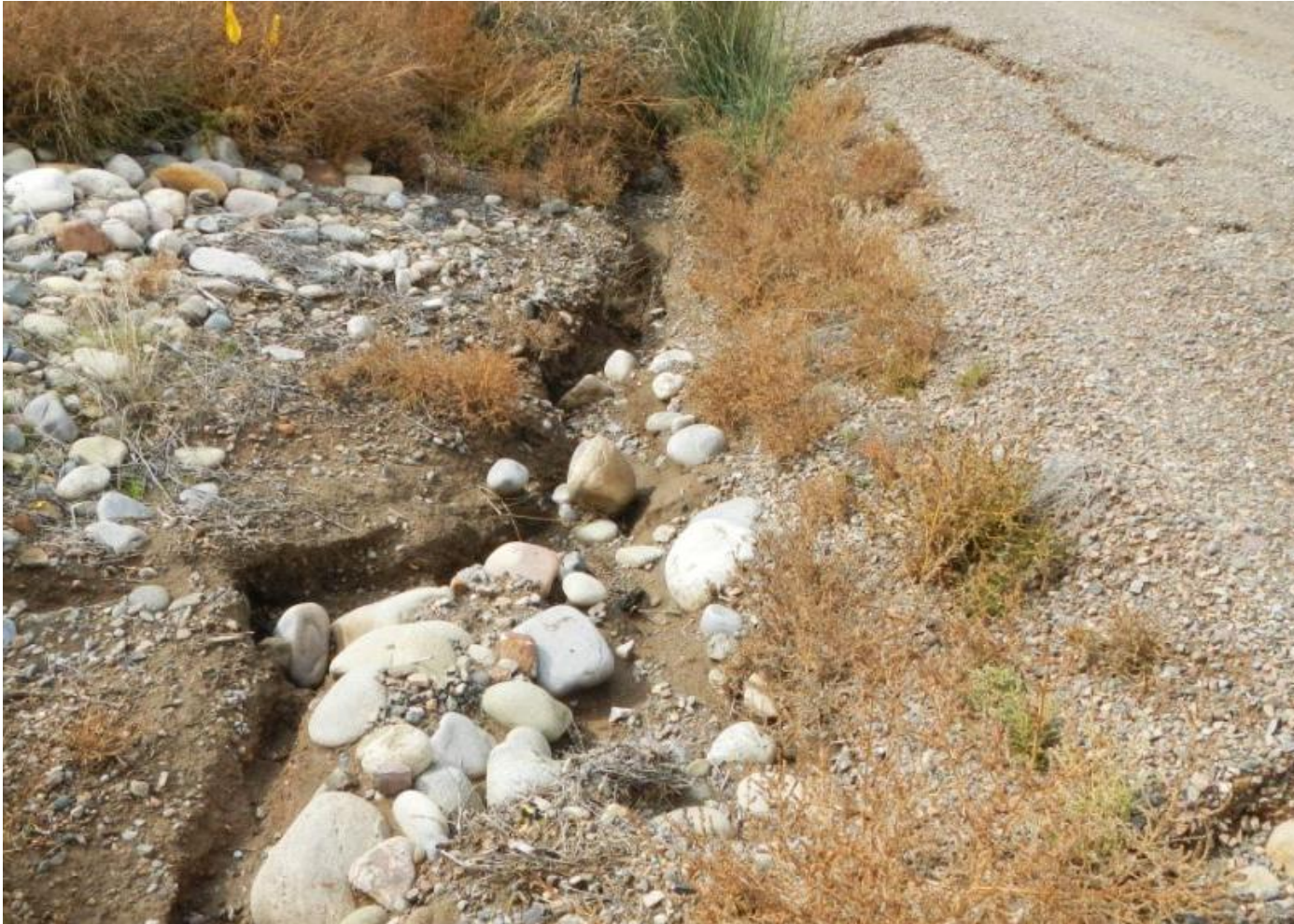
Photo 7. View of erosional channel forming along roadside and eroding road surface adjacent to the northern edge of the project area, facing downslope.
