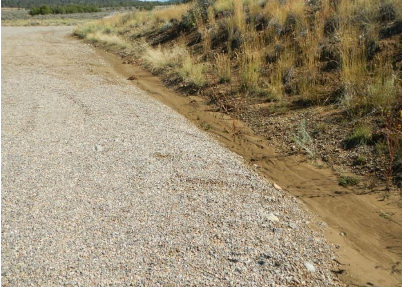
Photo 5. View of eastern edge of working area facing northward. Diversion is filling with sediment.
