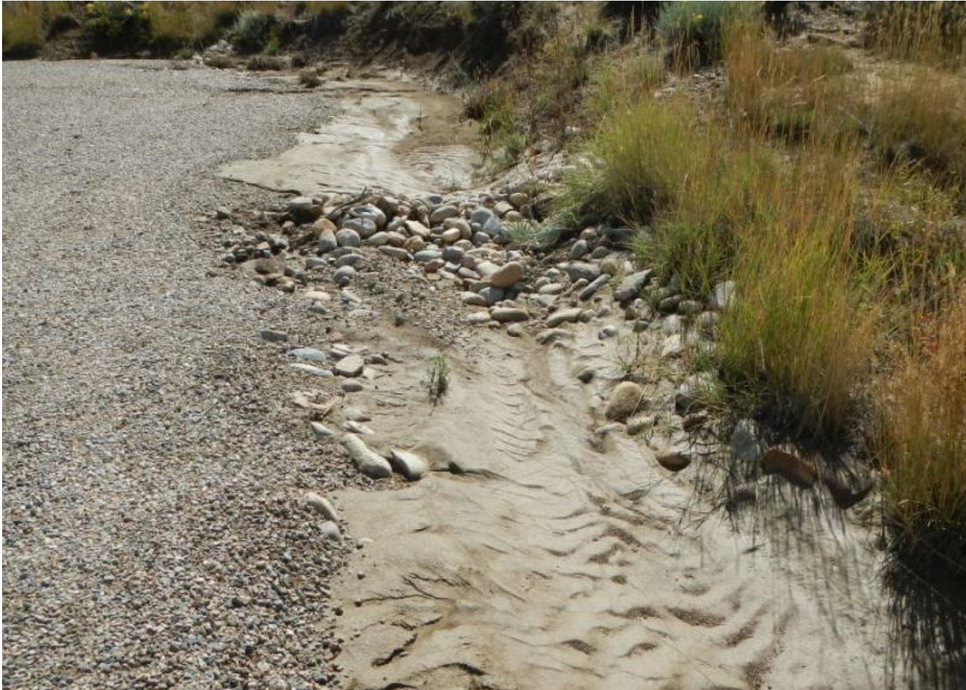
Photo 4. View of cobble BMPs and diversion filling with sediment along southern edge of working area.
