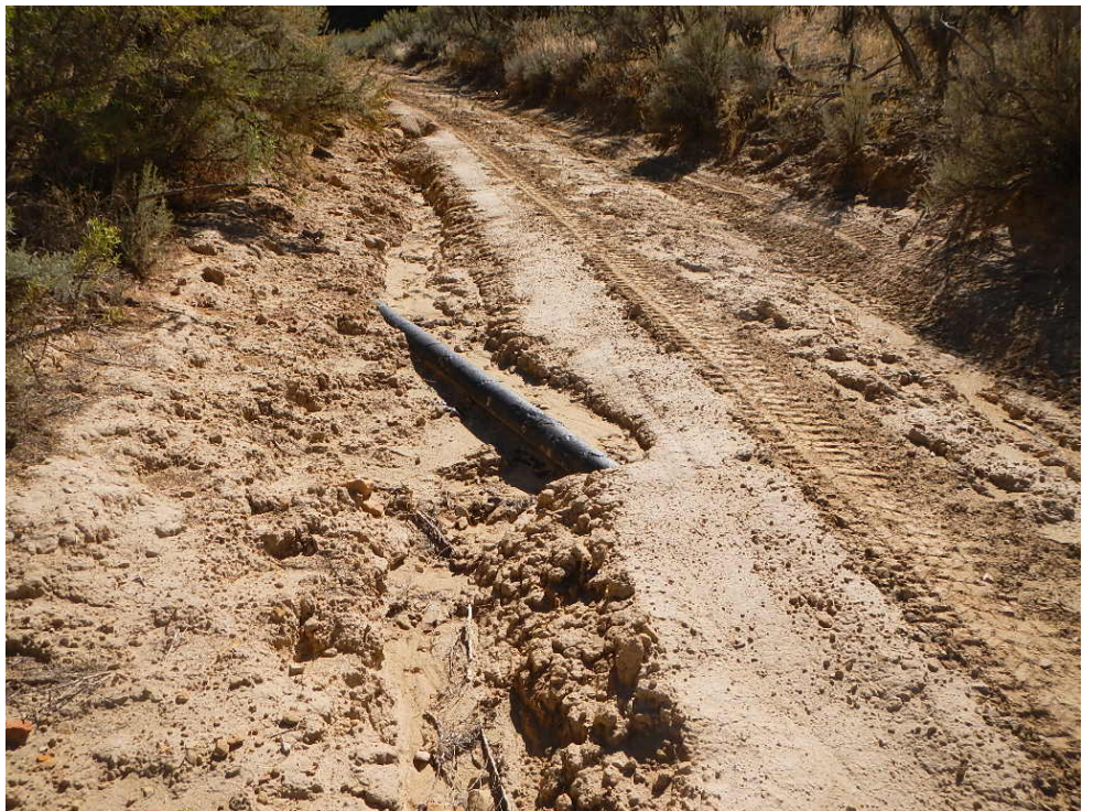
Exposed line from erosion of access road.
