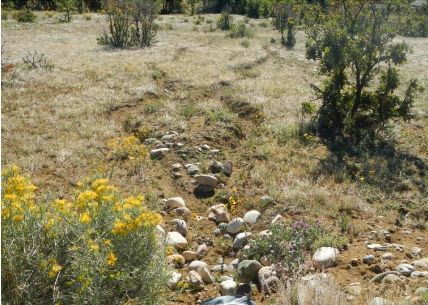
Photo 6. View of erosional channels approximately 2 feet wide and 2 feet deep are eroding into the hillside on the downstream side of the culvert shown in photos 4 and 5.
