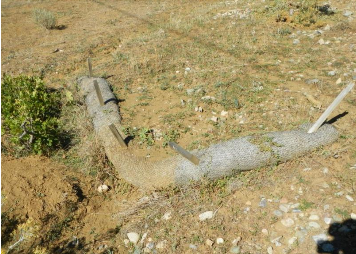
Photo 7. View of straw wattle on south side of the access road near the beginning of the access. Straw wattle is full of sediment, is eroding on the downstream side (on left) and stormwater flows appear to be bypassing the wattle and eroding around it (in background)
