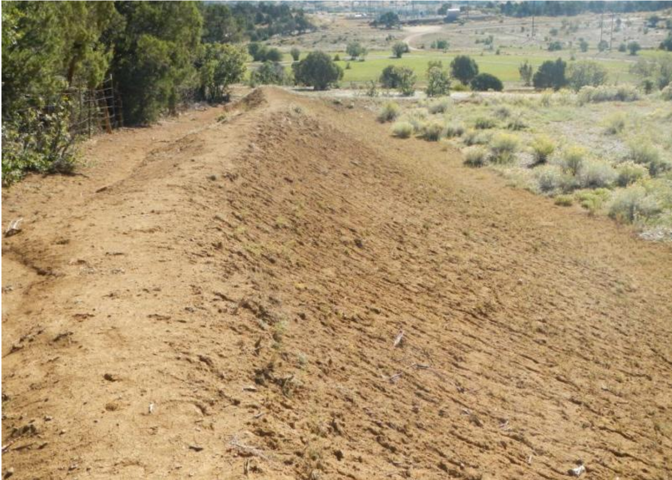
Photo 1. View of northern portion of project area from northwestern corner facing eastward. Rill erosion is occurring on the unvegetated cut slopes.
