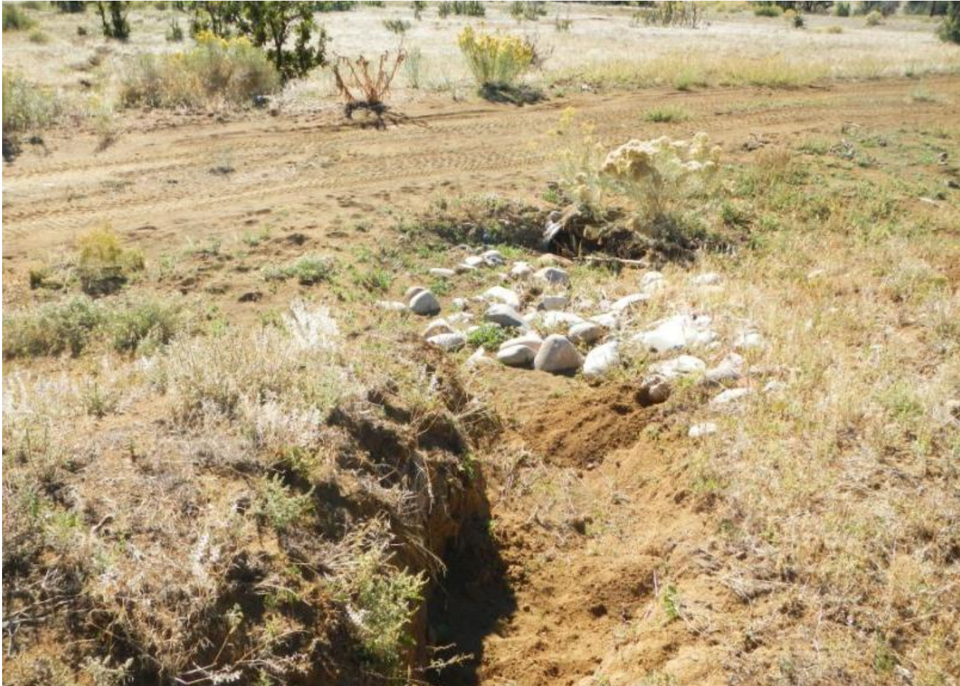
Photo 4. View of culvert along access road near the well pad entrance. Culvert is approximately 60 percent full of sediment and debris. It appears that stormwater flows frequently bypass the culvert and flow over the access road eroding the slope downstream (See photo 6).
