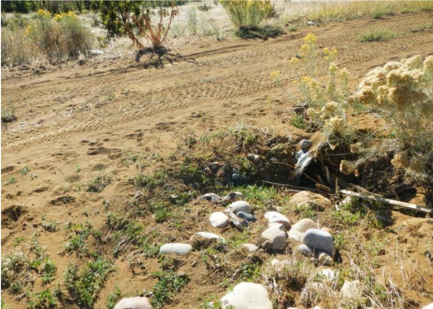
Photo 5. Closeup of culvert shown in Photo 4, showing that the culvert is large full of sediment and debris.
