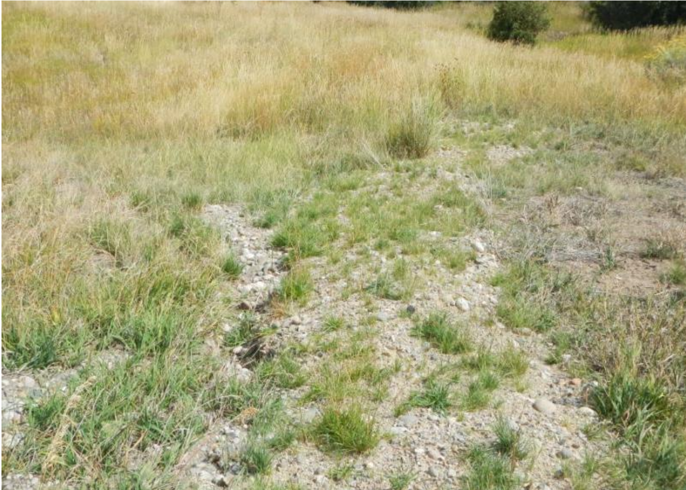
Photo 3. View of stormwater erosional channel that appears to have been filled and revegetated, facing downslope. Rilling is occurring on the sides of the channel as high energy water flows need BMPs to slow the water down.
