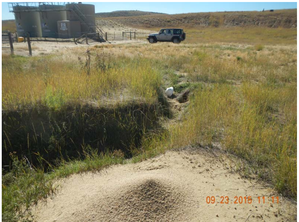
Erosion gully on north side of location. Hard hat for scale.
