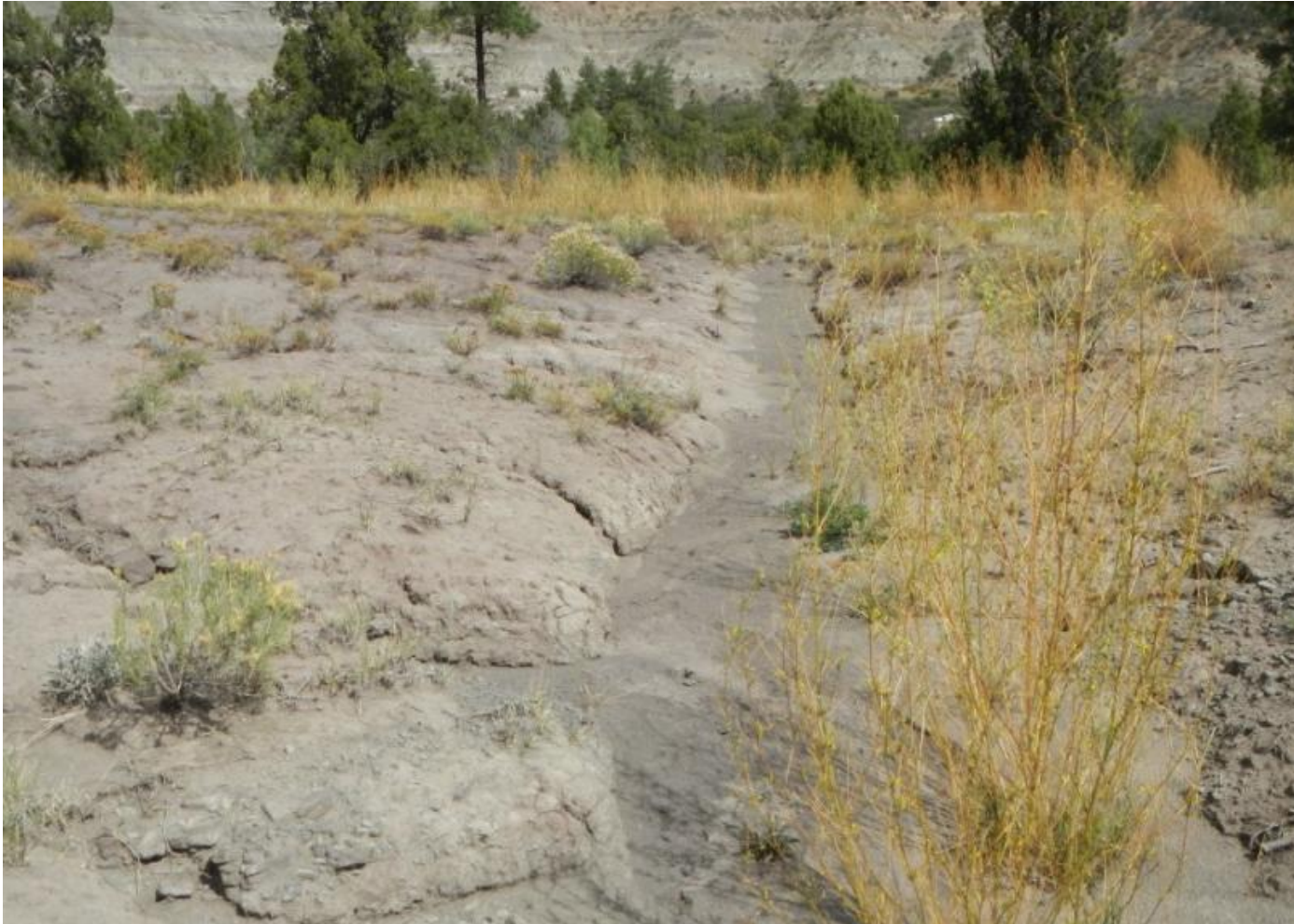
Photo 5. View of bar ditch along access road filled with sediment facing upstream toward the access road (northward).
