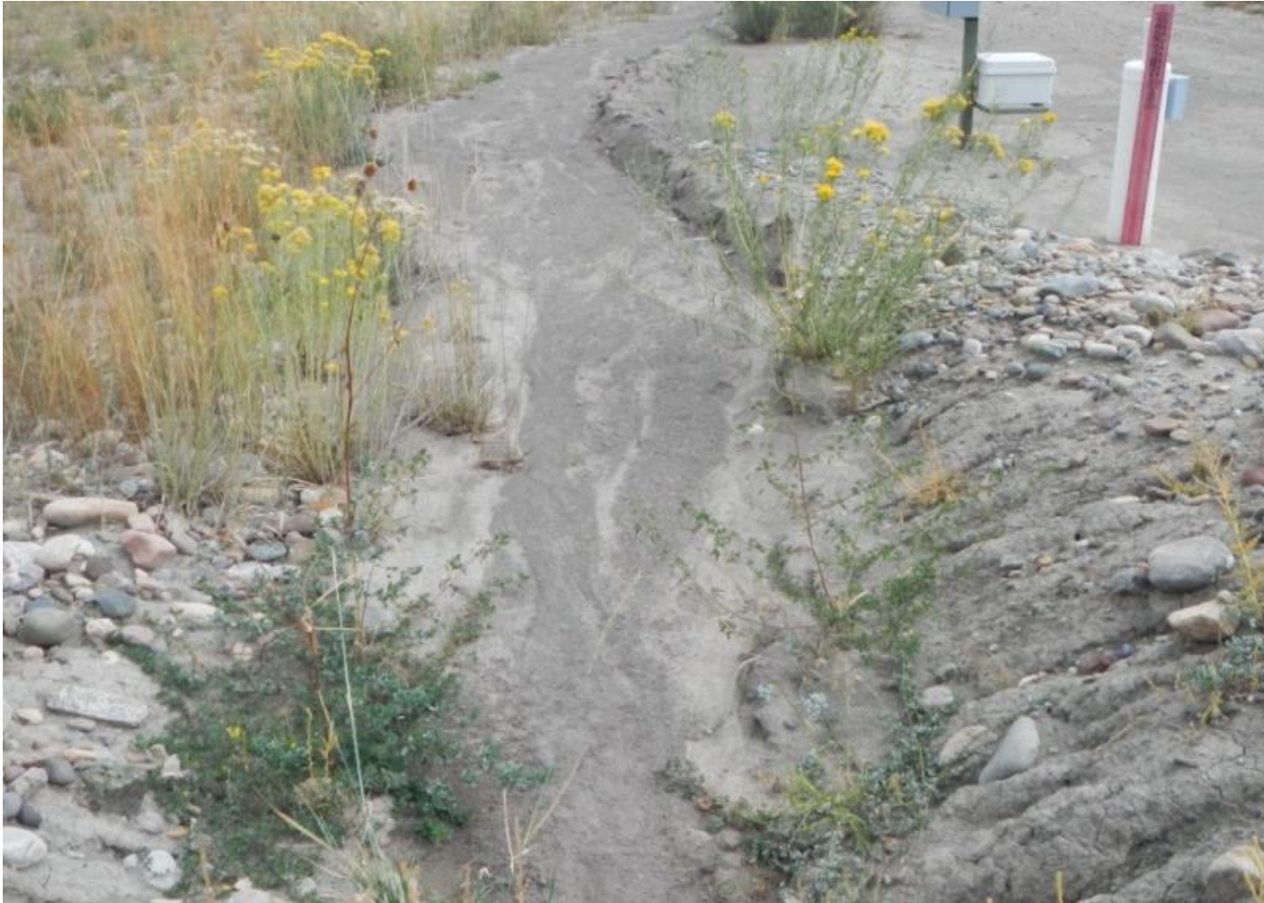
Photo 2. View of sediment filled diversion ditch on western and northern edges of the working area.
