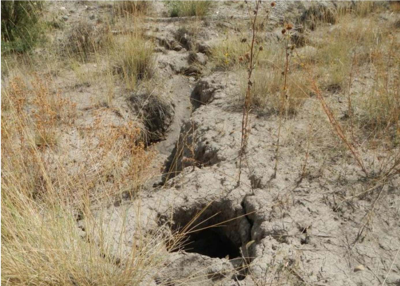
Photo 6. View of erosional channel and tunnelling in cut-slope along access , where it appears stormwater flows from the bar ditch have changed course and eroded through the fill slope. Photo facing downslope from top of hill.
