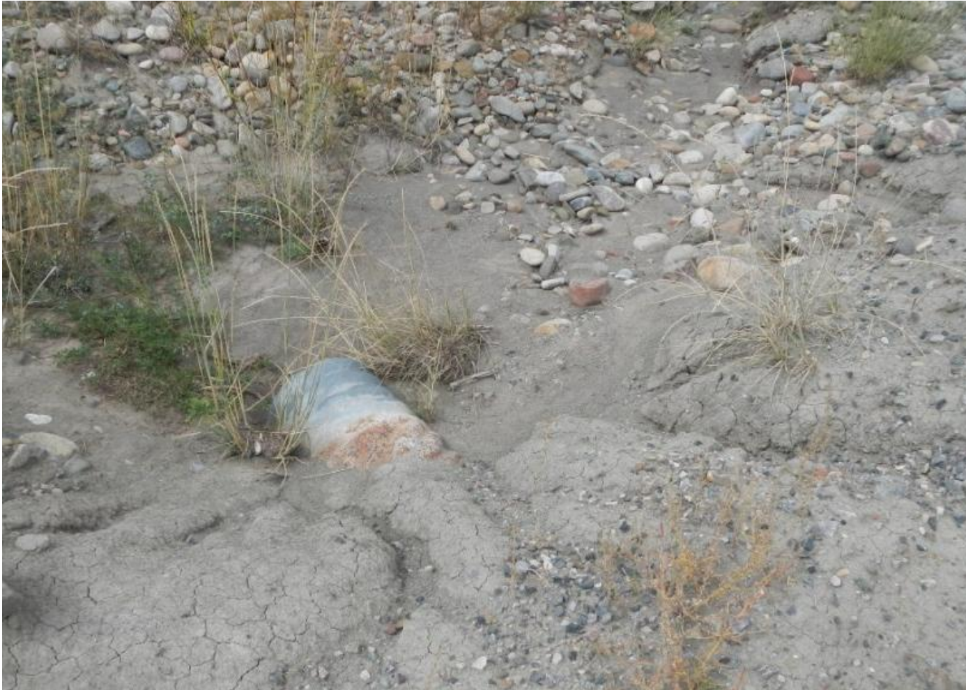
Photo 1. View of culvert inlet at entrance to well pad. Culvert is largely full of sediment, and erosion is occurring around the culvert.
