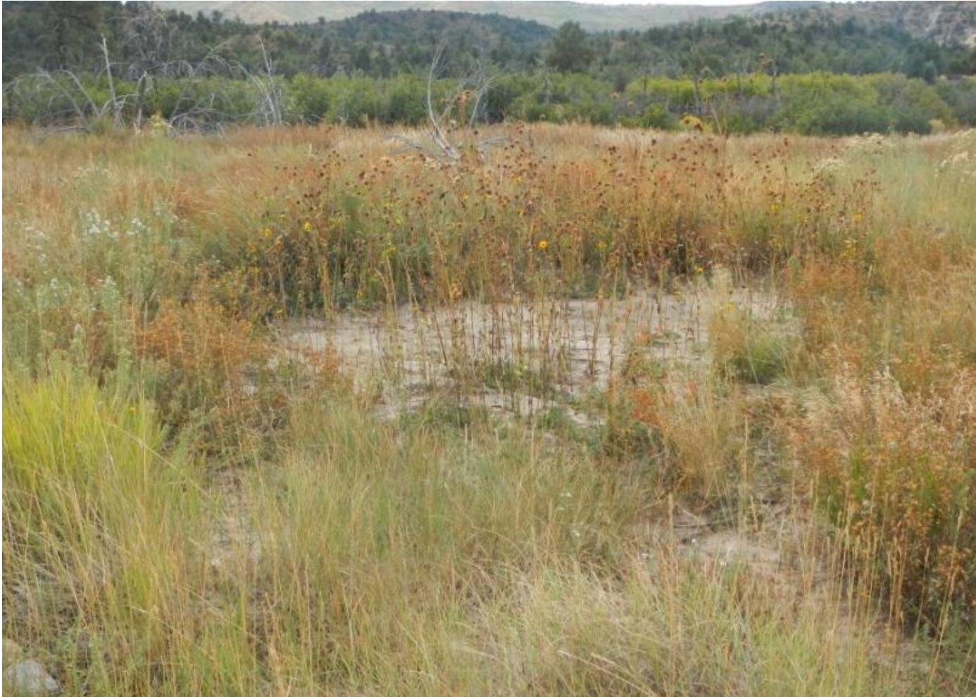
Photo 4. View of silt trap in eastern portion of project area. Silt trap is largely full of sediment and has breached an approximately 1.5 foot wide and deep channel in the supporting berm. Photo facing eastward from well pad.
