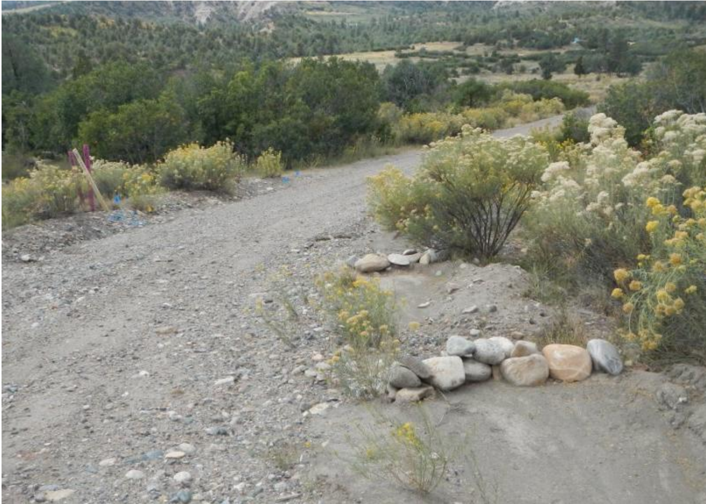
Photo 9. View of cobble filter dams along the access road that are filled with sediment, facing downslope (southward).
