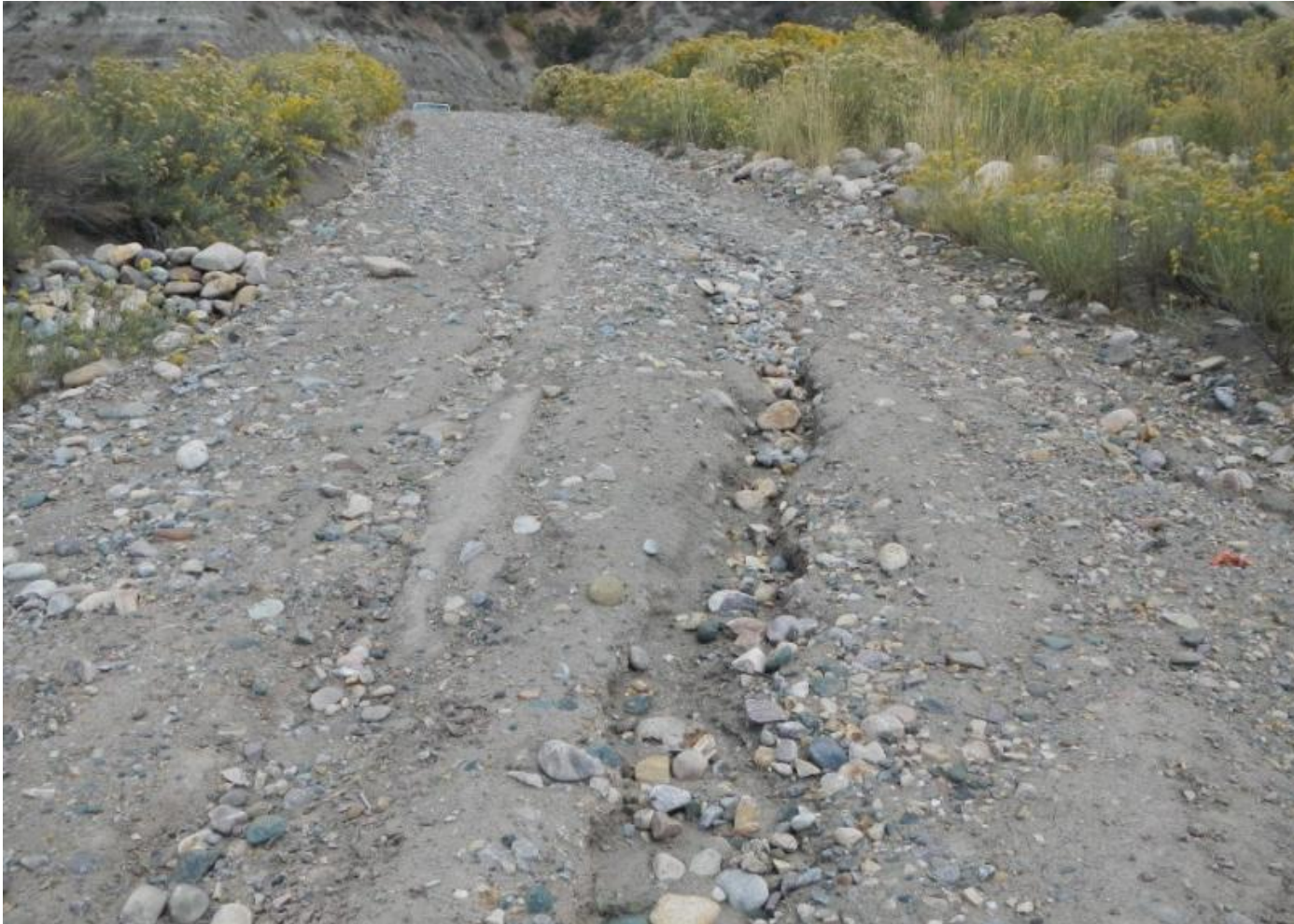
Photo 8. View of erosional channel on access road facing upslope toward well pad (northward).
