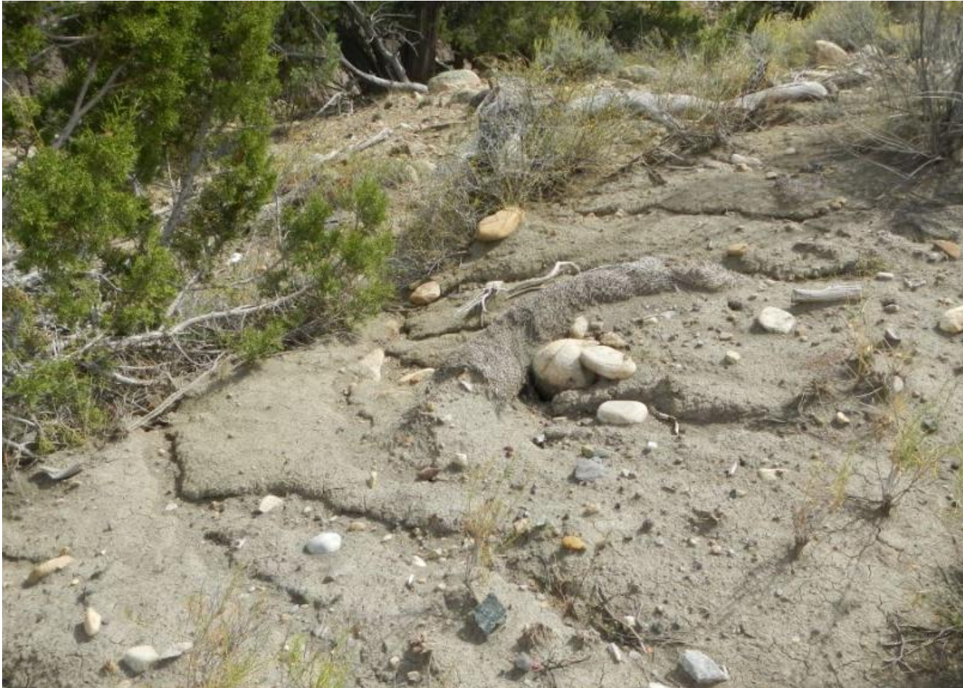
Photo 3. View of rills (approximate 5 to 8 inches deep) degraded straw wattle along eastern edge of project area.
