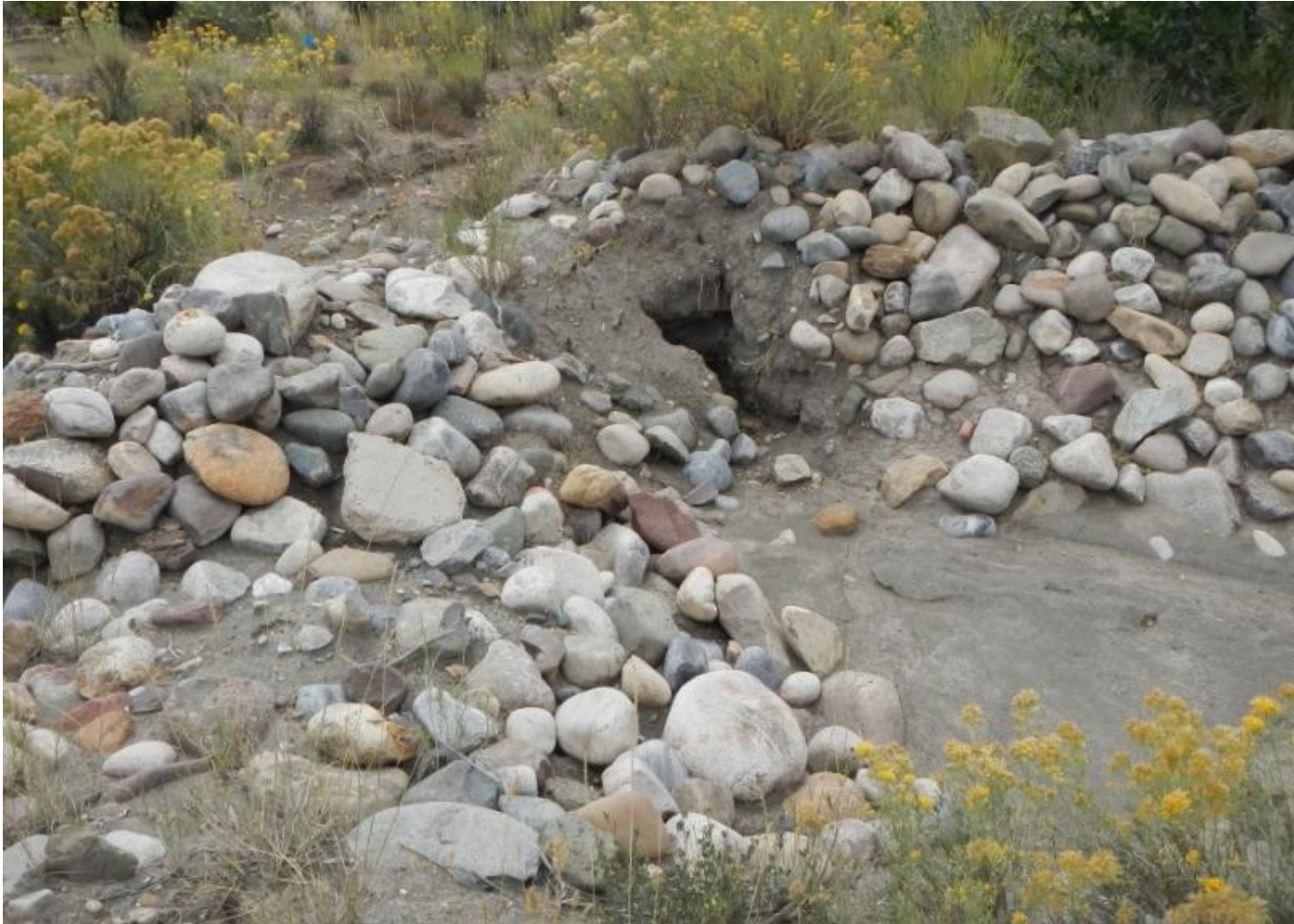
Photo 5. View of hole in silt trap where it appears stormwater and sediment flows during storm events. Located in the southern portion of the project area.
