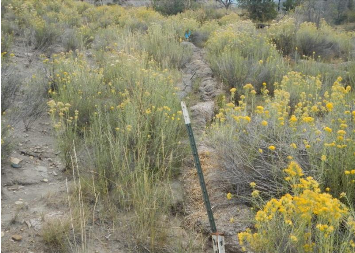
Photo 7. View of degraded straw bales and wattles in southern portion of project area.
