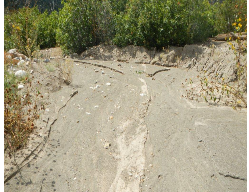
Photos 1 and 2. View of western portion of stormwater diversion channel that is full of sediment facing upstream (on left) and facing downstream (on right).
