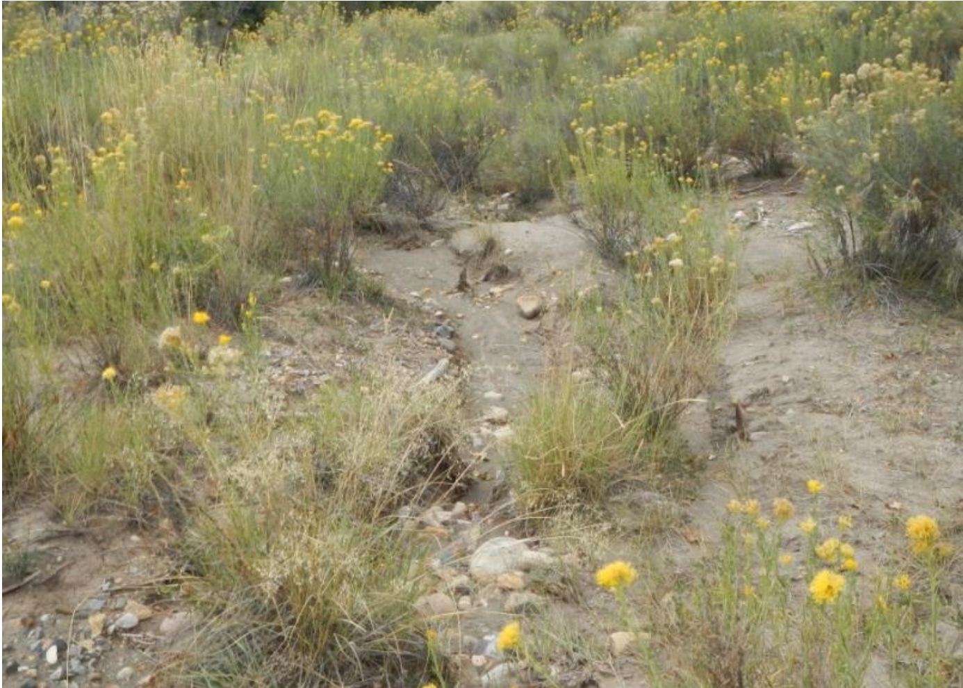
Photo 6. View of erosional channel downstream of eroded silt trap shown in Photo 5, facing downstream. Erosional channel is approximately 2 to 3 feet wide and 1 foot deep.
