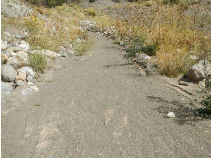
Photos 1 and 2. View of western portion of stormwater diversion channel that is full of sediment facing upstream (on left) and facing downstream (on right).
