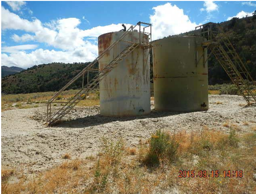
Tank berm not maintained – flat in areas
