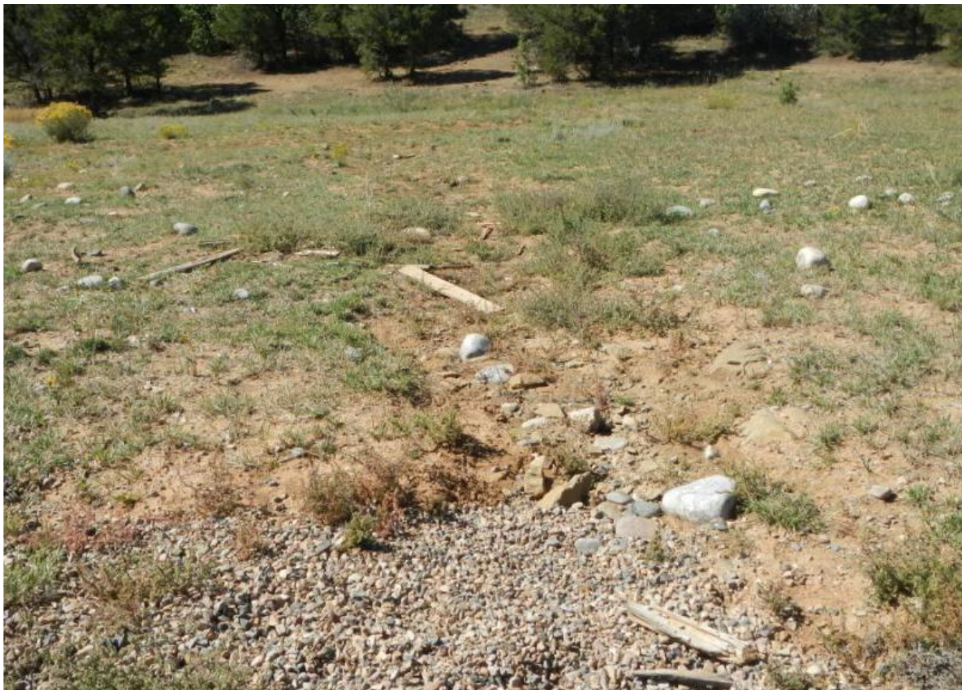
Photo 2. View of shallow erosional feature within western portion of project area. Small gravel/cobble has been placed here. This needs monitoring to make sure it does not worsen.
