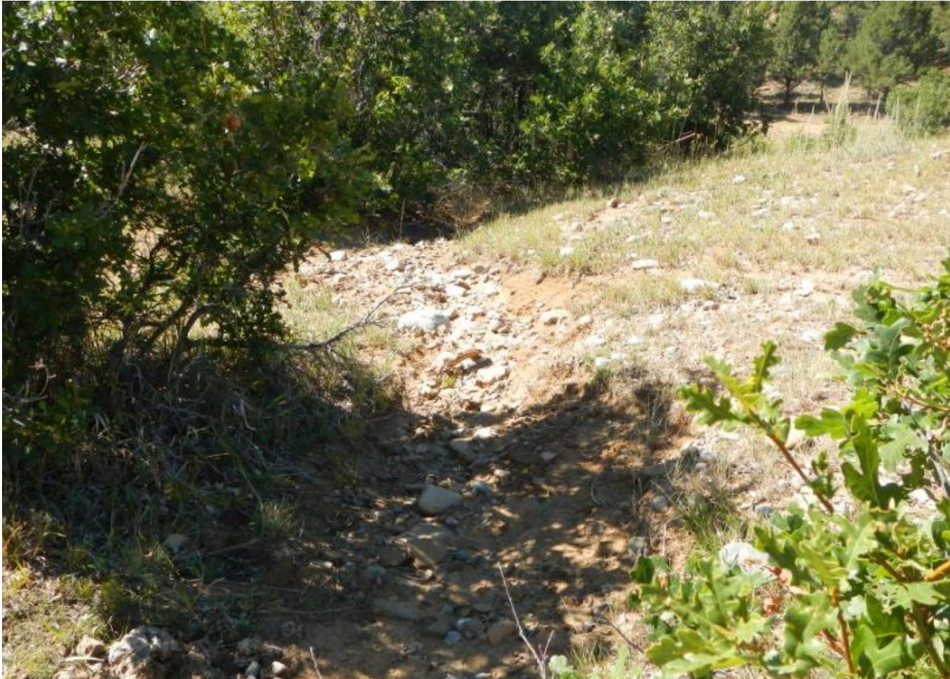
Photo 1. View of diversion channel in southern portion of project area, from southern edge of well pad facing westward. This should be monitored and BMPs applied if down-cutting worsens.
