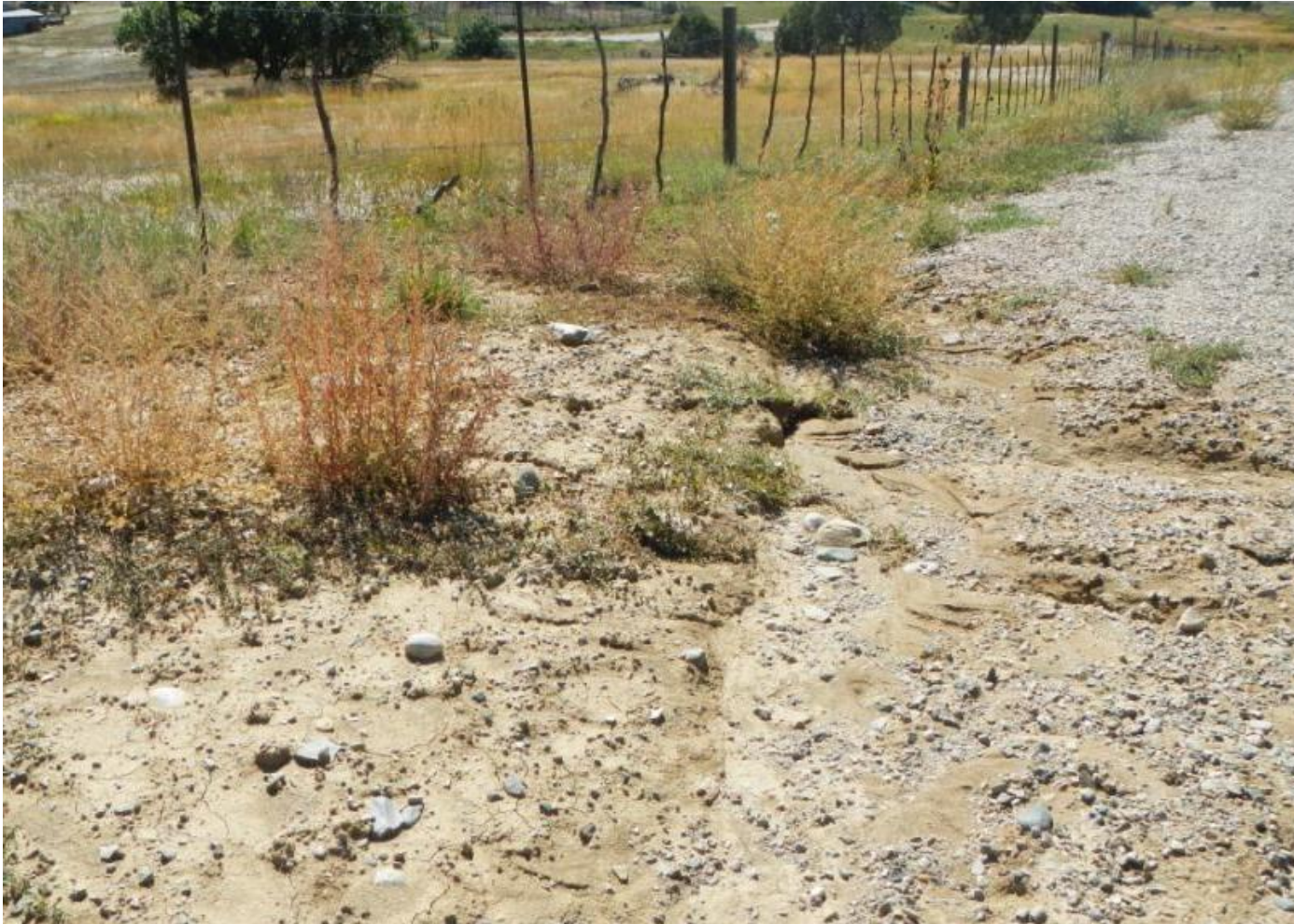
Photo 1. View of location in southern portion of well pad where concentrated stormwater flows appear to exit the well pad and flow into an erosional channel, from southern edge of well pad facing southwestward.
