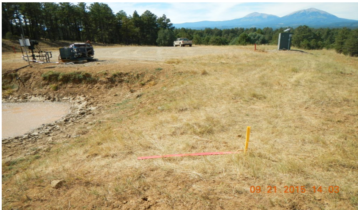
photo 3: Southeast side of the location facing northwest . Guy line marker has fallen over.
