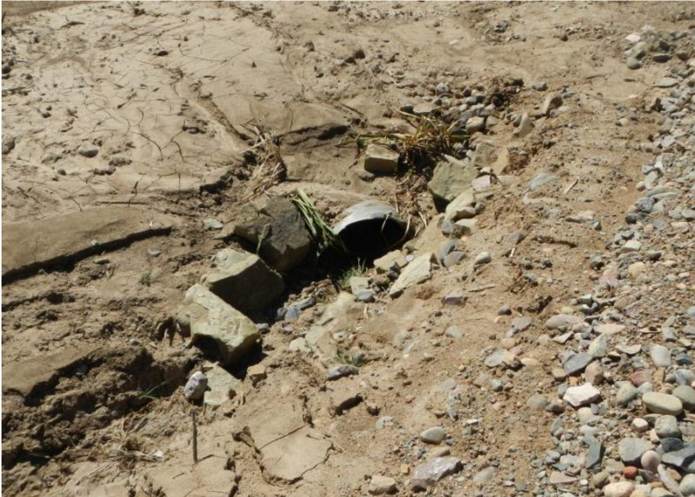
Photo 5. Closeup view of sediment filled culvert on south side of access road, along middle portion of access road.
