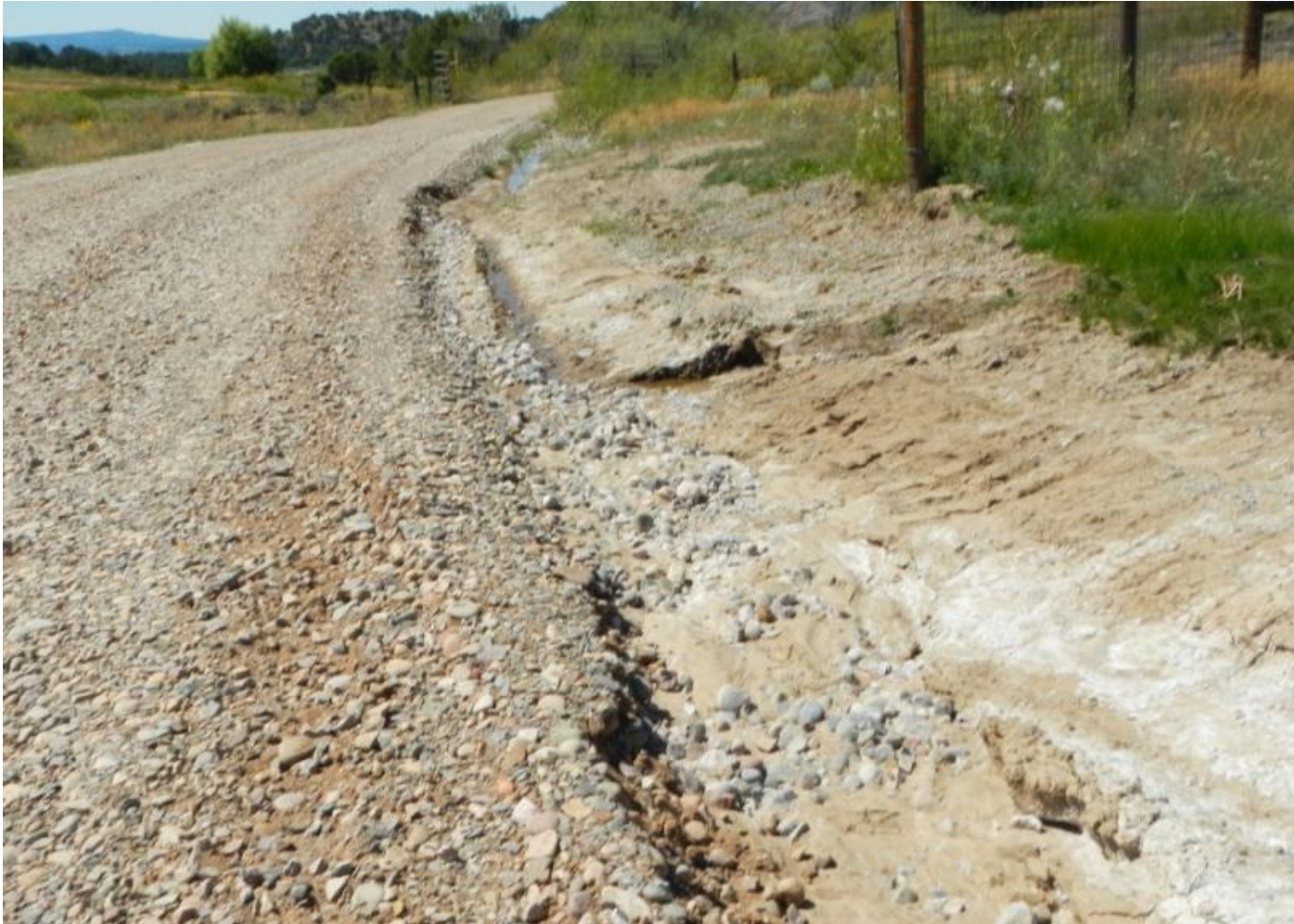
Photo 6. View of erosional channel forming along northern edge of the access road, along middle portion of access road.
