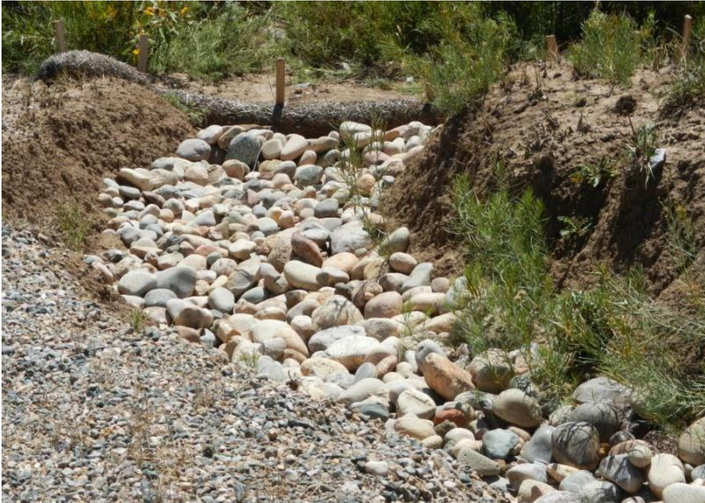
Photo 12. View of cobble armored erosional channel and wattle in southeastern corner of project area facing downstream.
