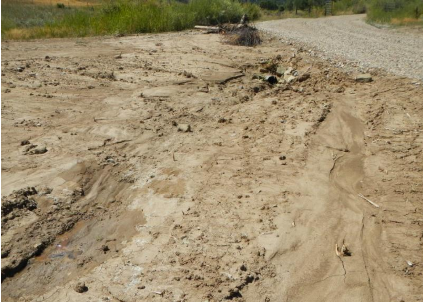
Photo 4. View of stormwater erosion on bare area south of access draining toward a culvert, along middle portion of access road.
