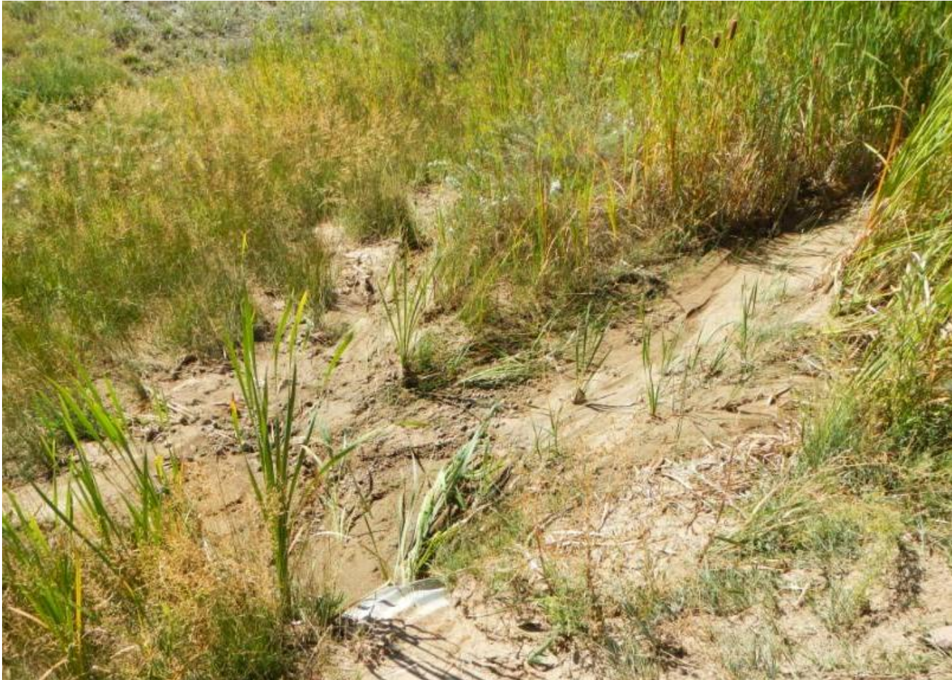
Photo 9. View of sediment deposition and transport at culvert outlet along access road.
