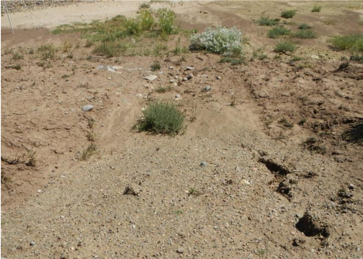
Photo 10. View of erosion along western cut-slope facing downslope.
