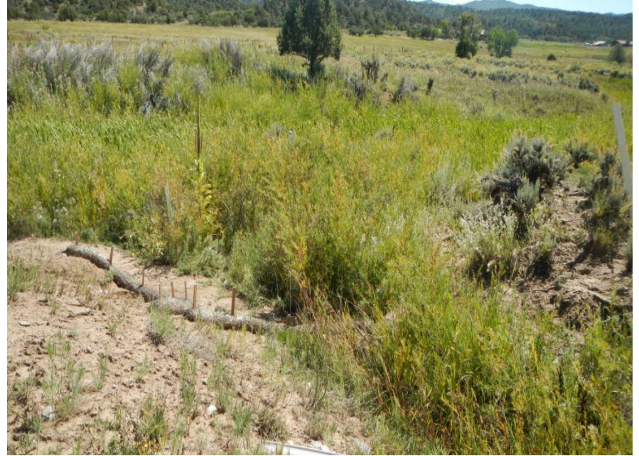
Photos 13 and 14. View of erosional channel forming off of the southern edge of the well pad (on left) and wattle placed in channel facing downstream (on right). Stormwater BMPs do not appear sufficient here as sediment appears to be running off the well pad down this channel toward wetlands and stream adjacent to project area.
