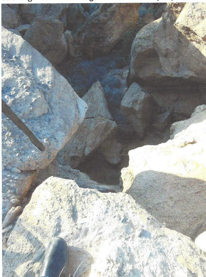
Looking down over edge of Butte into spill path
