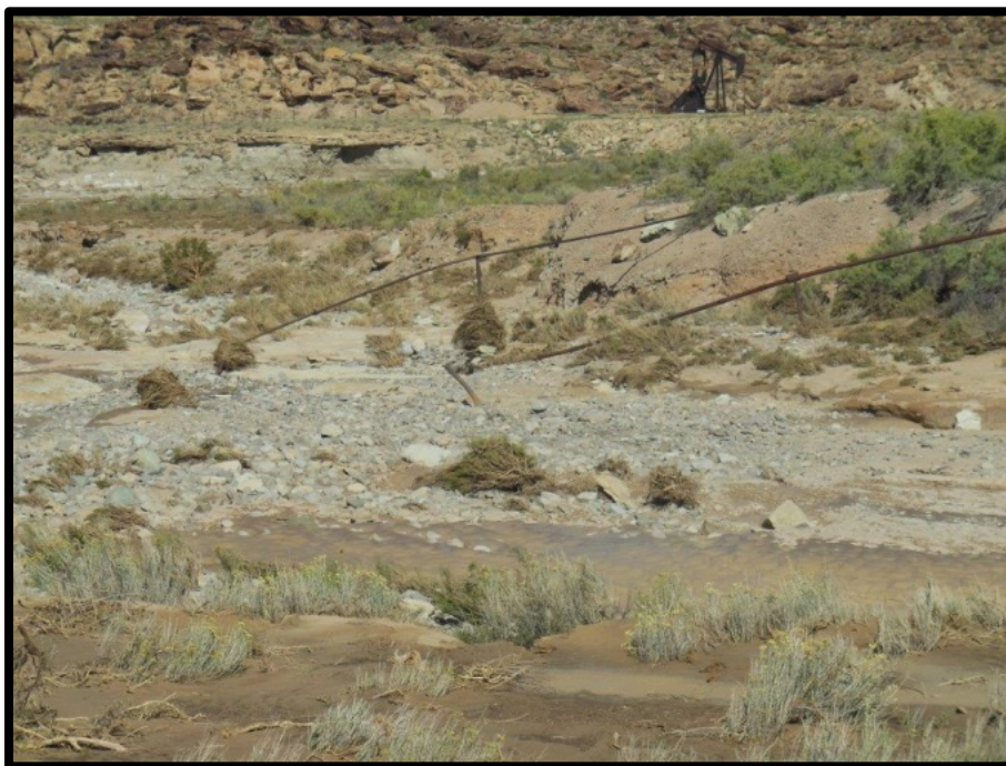
9/18/13: View of destroyed pipelines crossing washing near Spill #1
