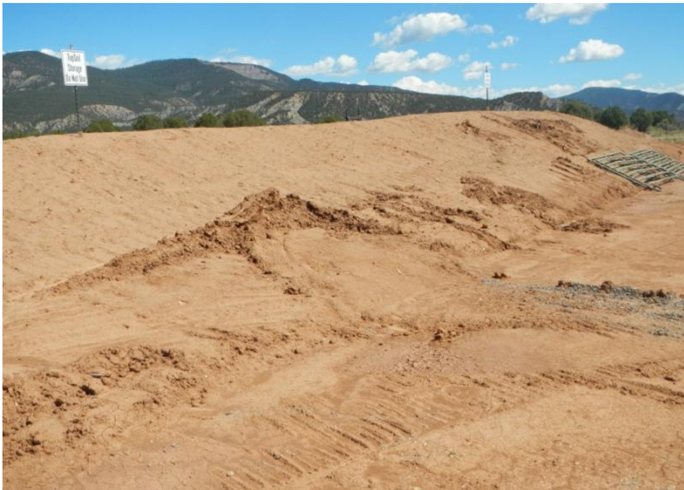
Photo 2. View of topsoil stockpile in northern portion of project area. Straw wattles present along northern edge. No stormwater controls for topsoil on well pad side. If interim reclamation isn't completed within the next month, then the entire topsoil stockpile will need stabilization.
