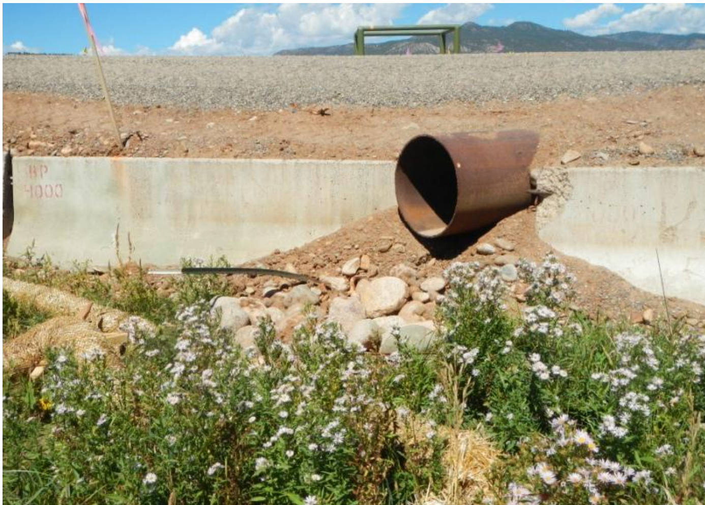
Photo 1. View of culvert outlet downstream of project area. No significant stormwater erosion is occurring here at this time.
