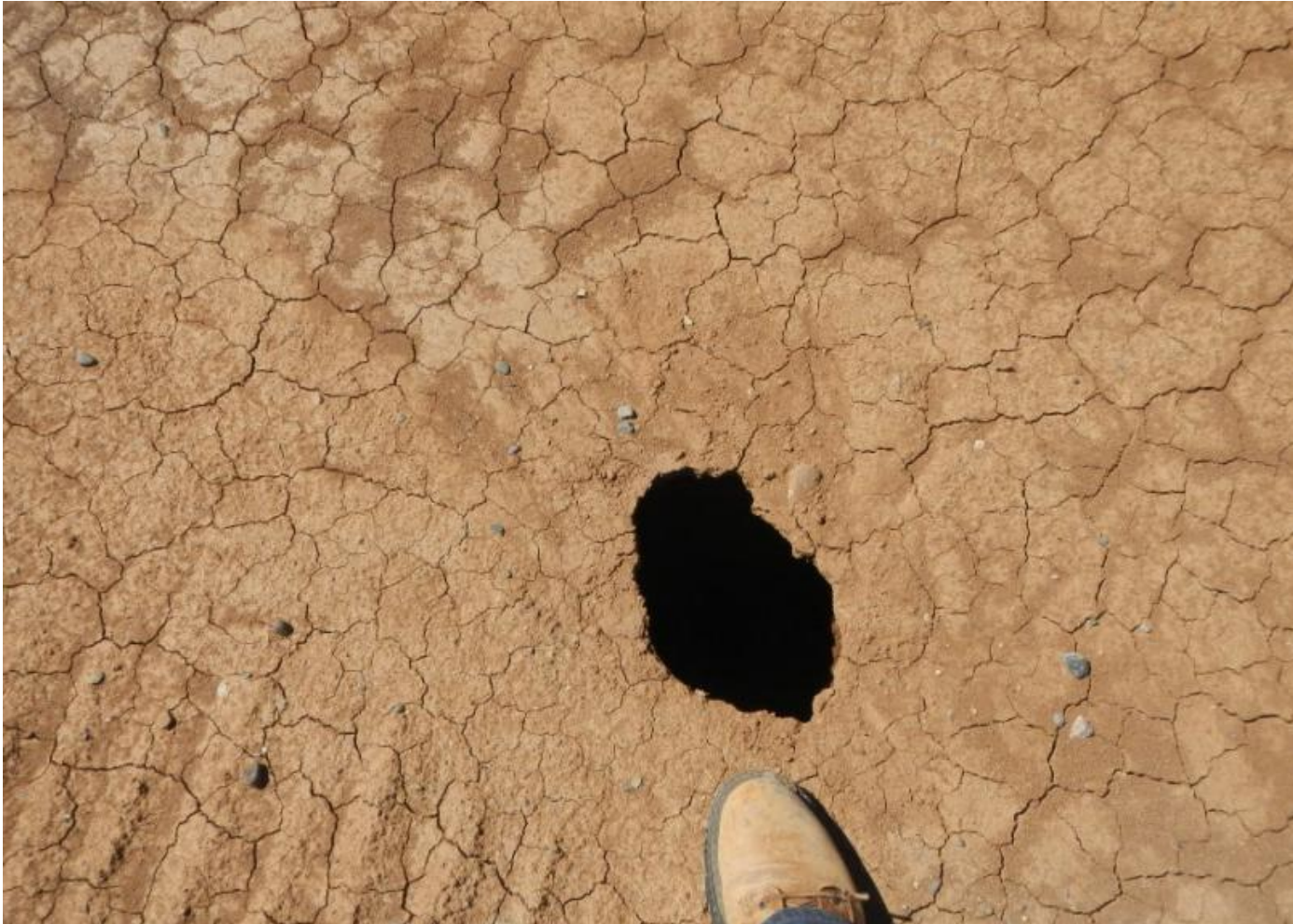
Photo 3. View of hole in well pad surface approximately 8 inches wide and 18 inches deep, that needs repair.
