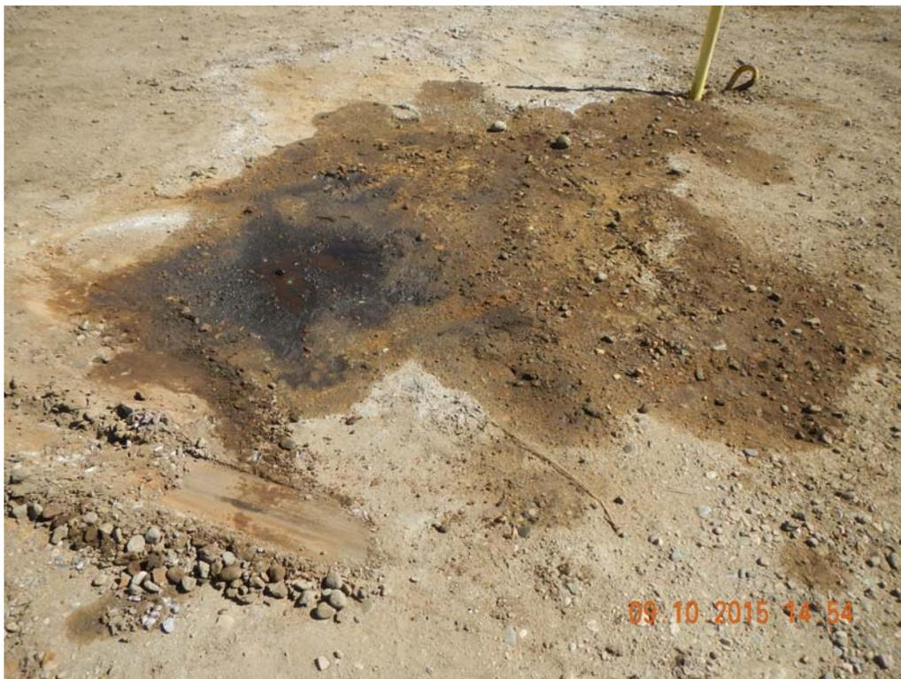
Stained soil at wellhead, fluid in cellar.
