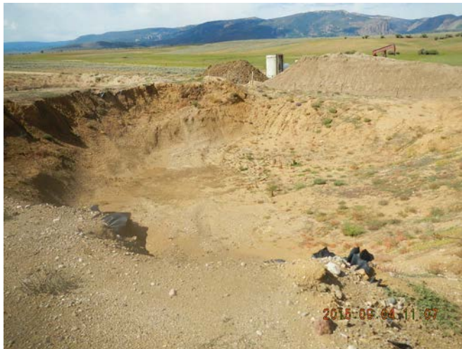
Pit Facility 115241- Pit bottom appeared to be moist with some vegetation growth. Material has sloughed from the sides or upper portion of the pit. Surface water runoff from the main Facility is controlled via a ditch was constructed along the north side of the Pit Complex. Pit not netted.
