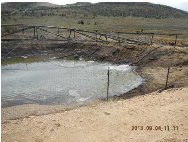
Pit Facility 112265- Fluid in pit app 15-20' below berm. Visual signs of hydrocarbons on fluid surface (10% of surface), netted but compromised with holes, visual staining of hydrocarbons along sides of pit. Used oil absorbent booms along east bank of pit. Fluids from Pit Facility 112266 were being transferred via a pump with 2-inch hose (estimated 60-80 gallons per minute)
