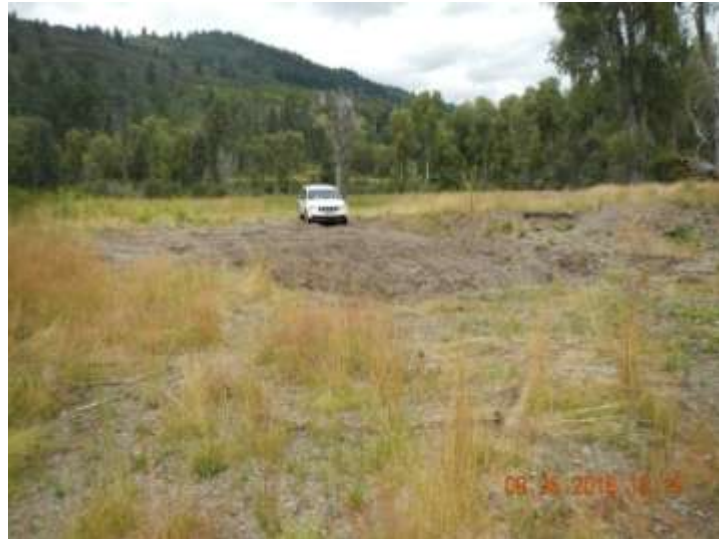
Gravel Pit – Approximate area of “low point” in historic pipeline. Slight hydrocarbon odor and what appeared to be stained soils present. A sample was collected from this material for analysis.
