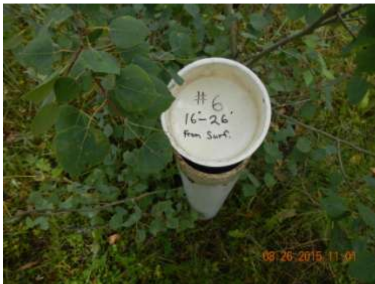
MW #6 – 4" PVC pipe approximately 2' above ground surface. Hydrocarbon odors present. Surface water located approximately 20' to the south does not appear to be impacted.
