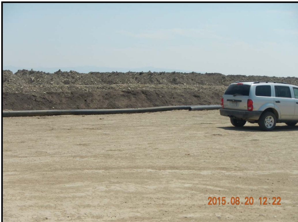
Stockpiles / Land Treatment Cells. Looking north. Piping that will not be used should be removed.
