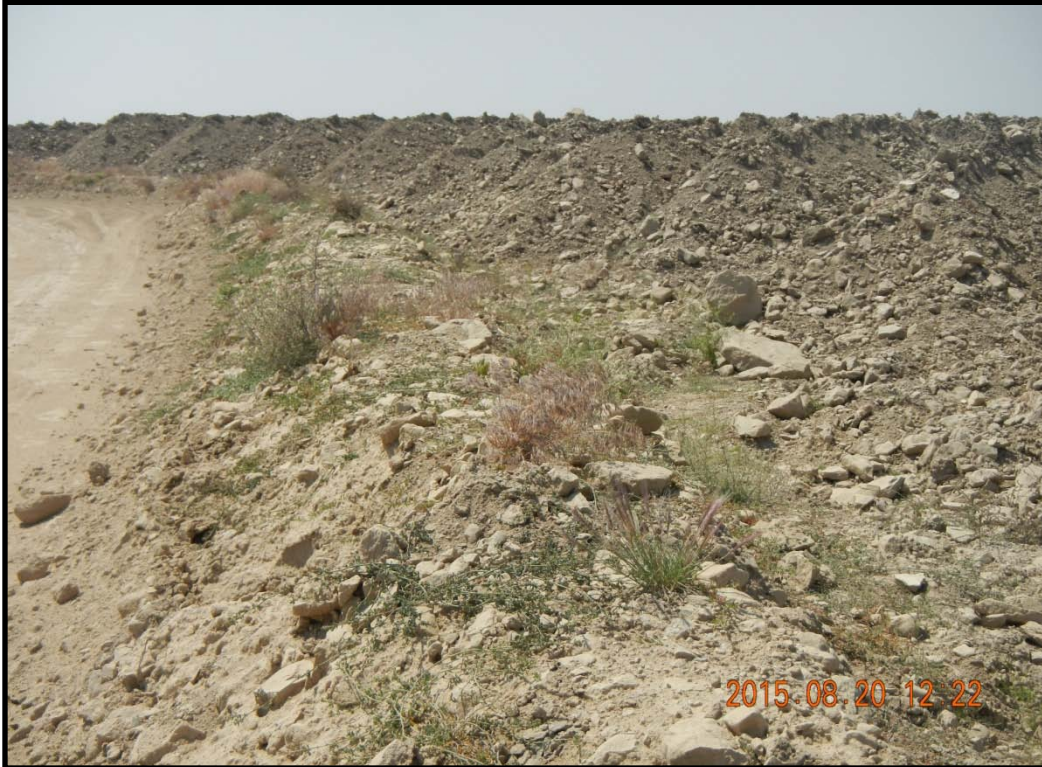
Treatment cells are bermed but not lined.
