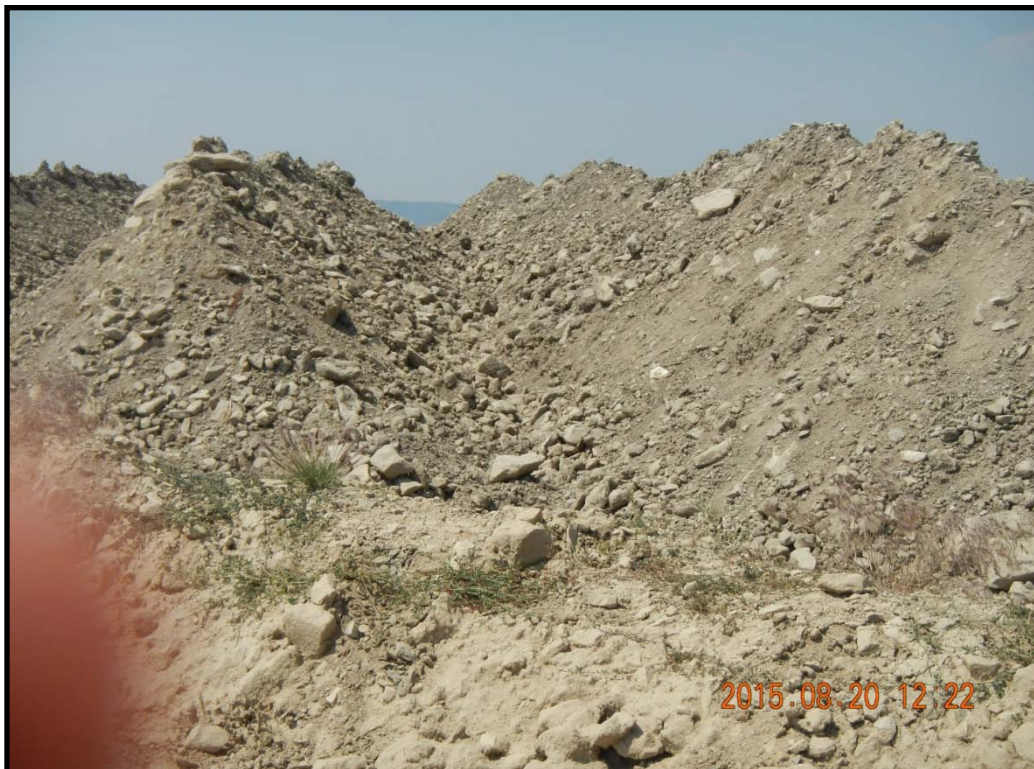
Treated soil in Windrows 6 feet or higher. According to Linn Energy representatives, this soil is moved about twice a year to improve remediation. Fertilized or other additive may be incorporated to the soil.
