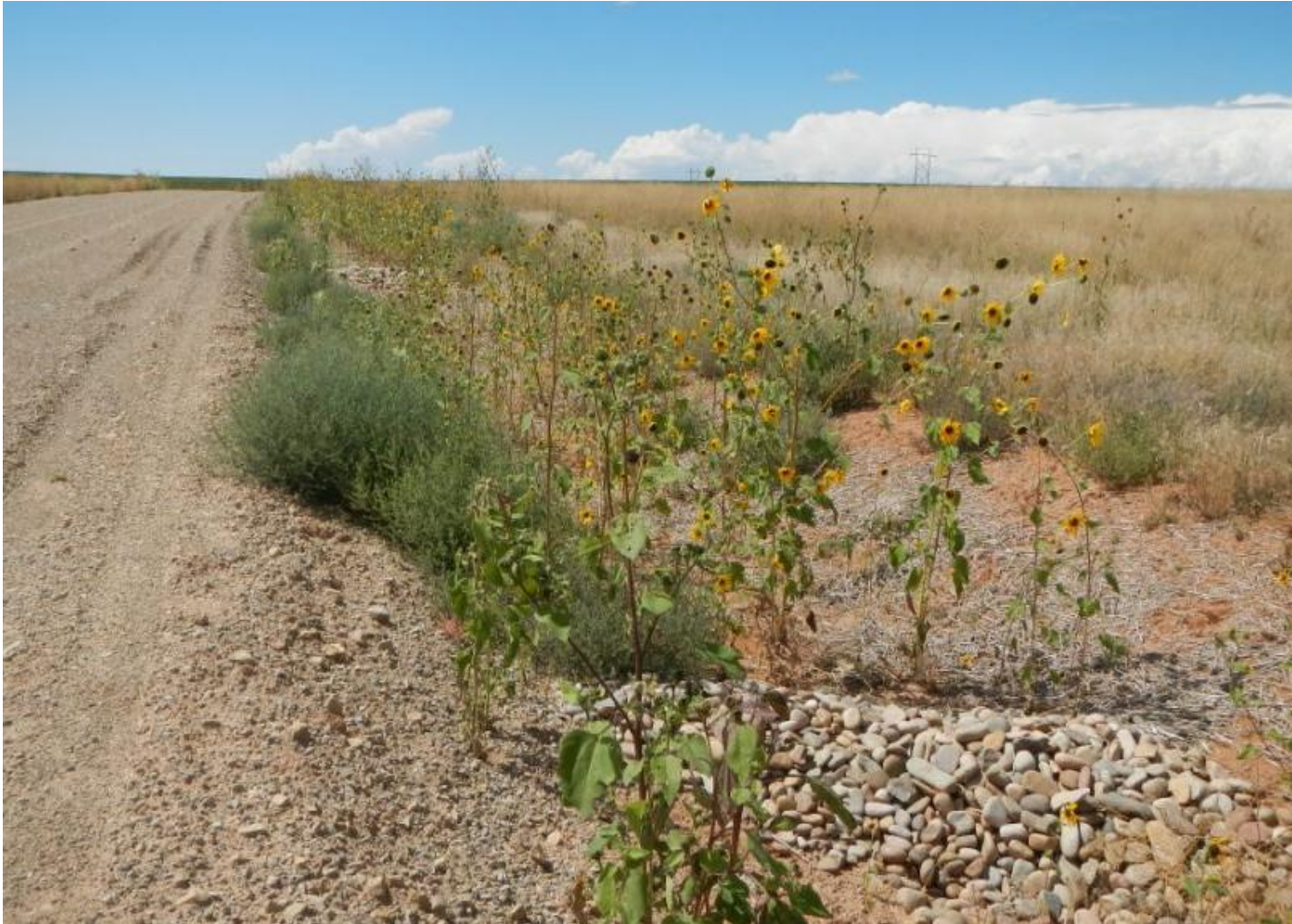
Photo 3. View of the northern portion of the access road from the well pad entrance facing westward. Cobble BMPs and straw mulch appear to be functioning.
