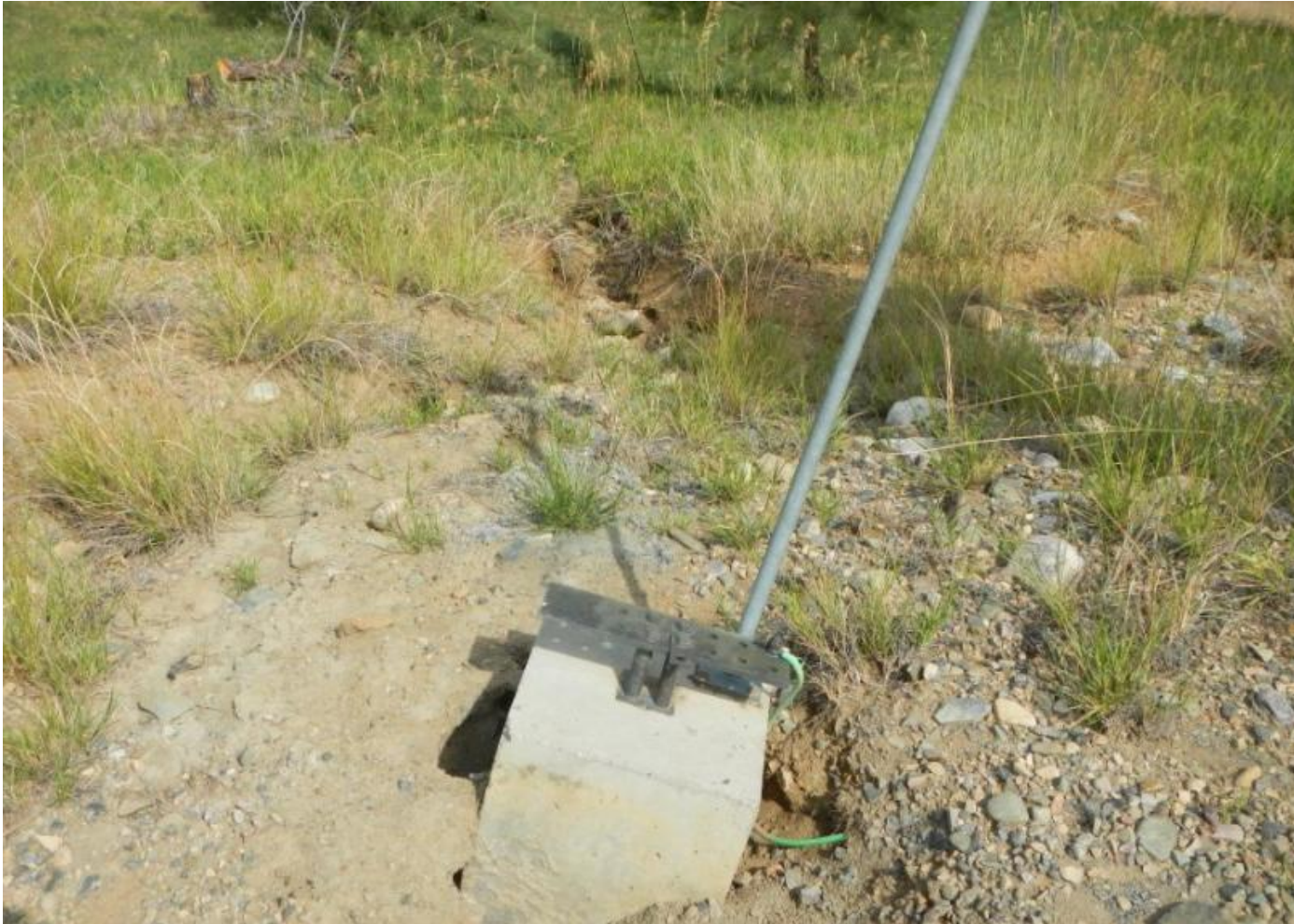
Photo 4. View of stormwater erosion occurring around project facilities in the eastern portion of the project area. This should be stabilized.
