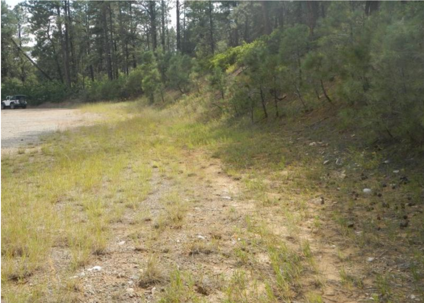
Photo 3. View of western portion of project area from northwestern corner facing southward. Vegetation on slopes and flat surface appear to be effectively stabilizing the cut-slope.
