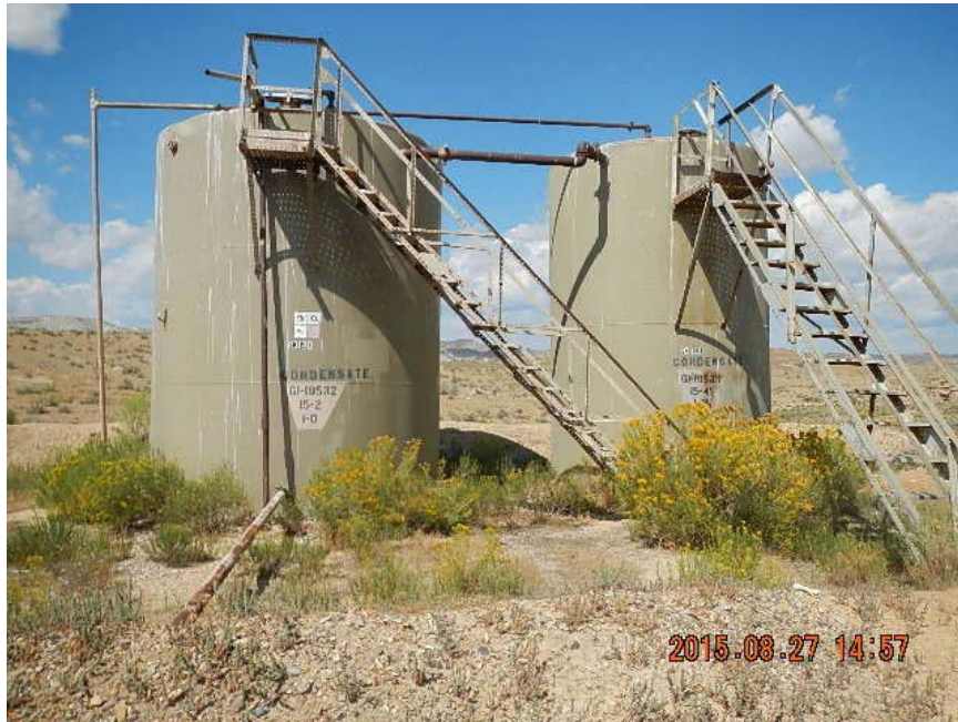
Tanks – not labeled/no battery sign
