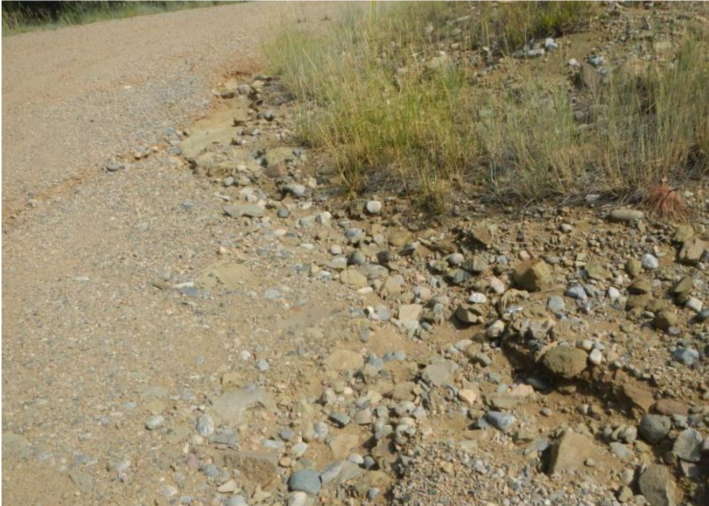
Photo 2. Another view of the erosional channel shown in Photo 1, and erosion on access road surface.
