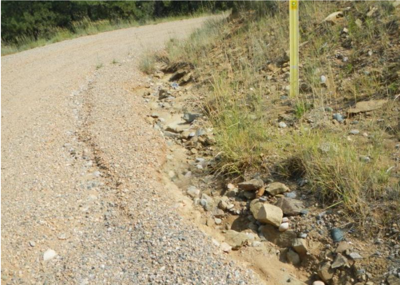
Photo 1. View of stormwater erosion along the access road and along the road surface. Erosional channel is approximately 2 to 3 feet wide and 18 inches deep.
