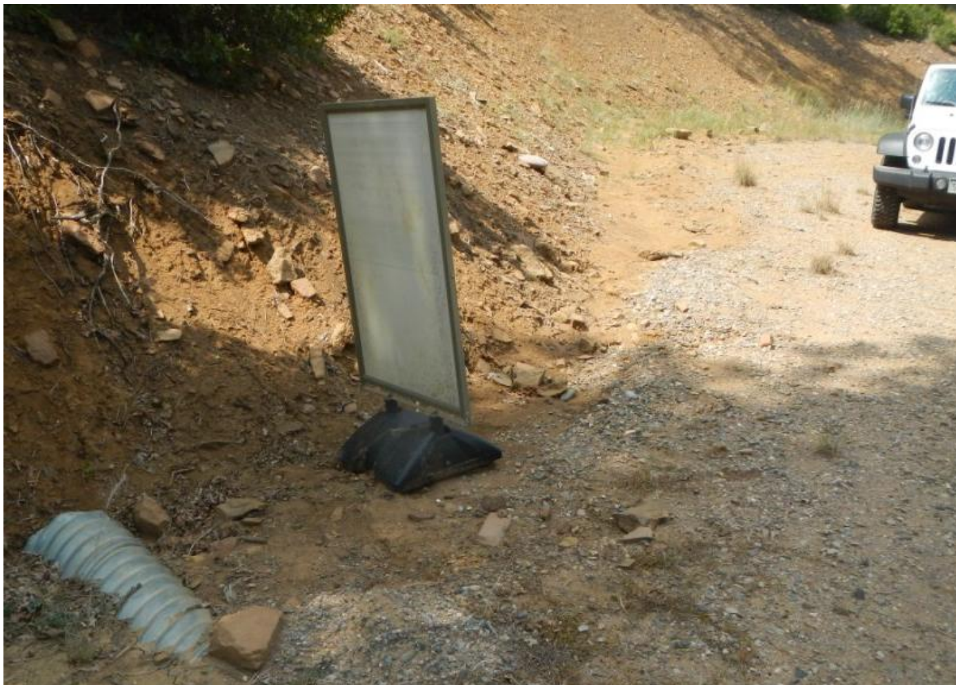
Photo 2. View of culvert and diversion that is full of sediment and not large enough for capacity. It appears that stormwater flows circumvent the culvert here and flow over the road, eroding the fill slope at the culvert outlet shown in Photo 1.
