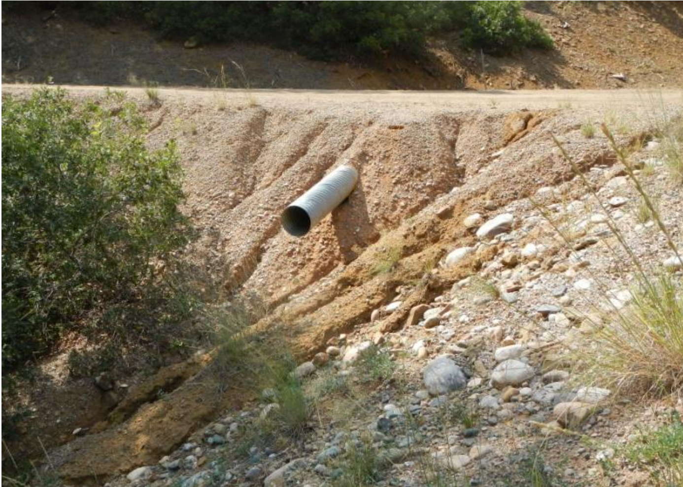
Photo 1. View of erosion at culvert outlet facing toward access road at entrance. Erosional channels are approximately 1 to 2 feet wide and deep.
