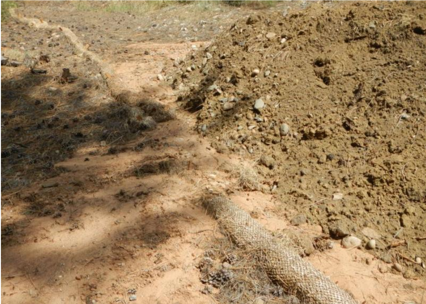
Photo 4. View of location on northern edge of project area where sediment appears to be flowing over wattle and needs maintenance.
