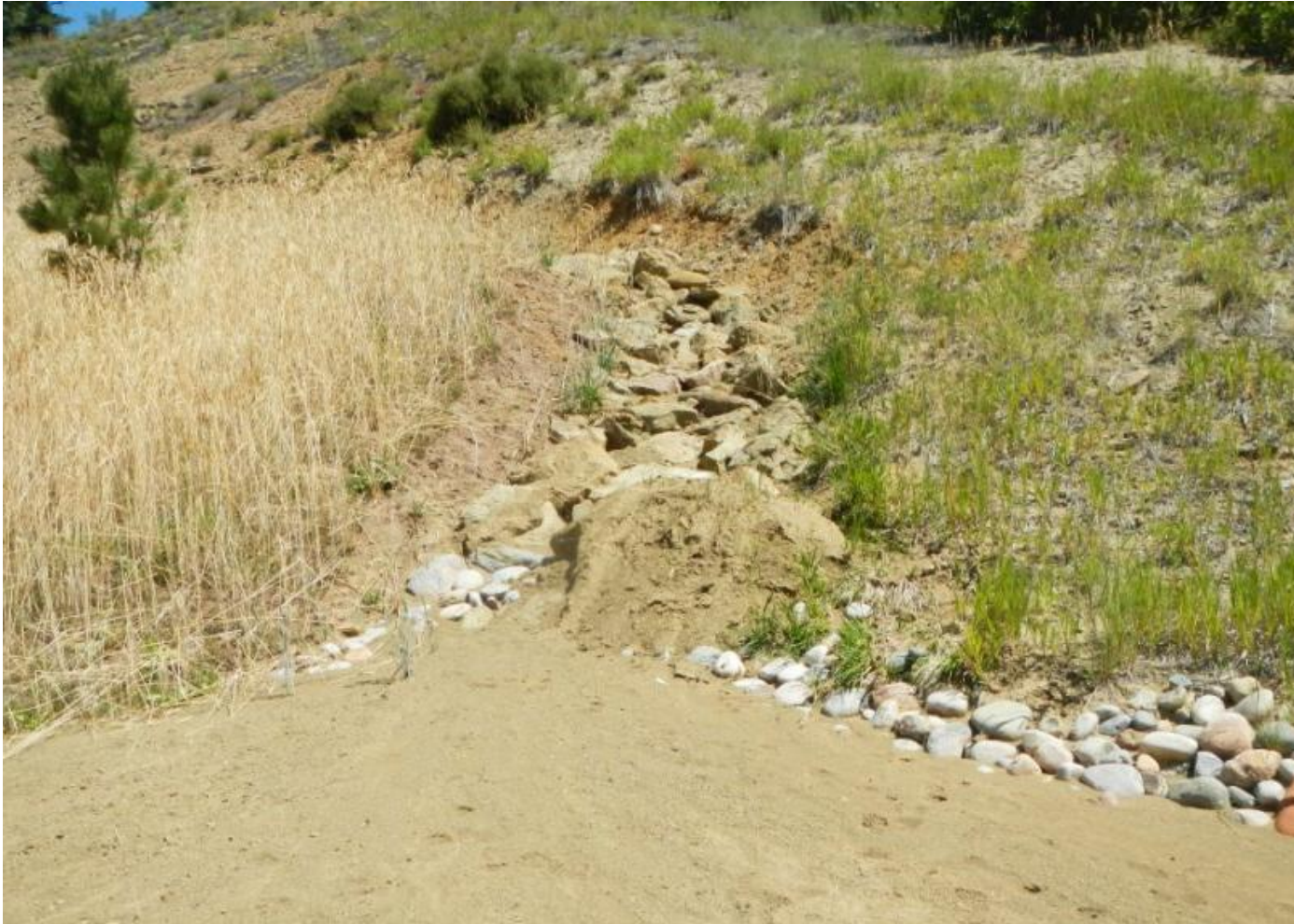
Photo 3. View of cut-slope diversion facing up-slope. Sediment plume in foreground appears to have been carried from the cut-slope and deposited here. This needs to be cleaned for continued functioning of the diversion.
