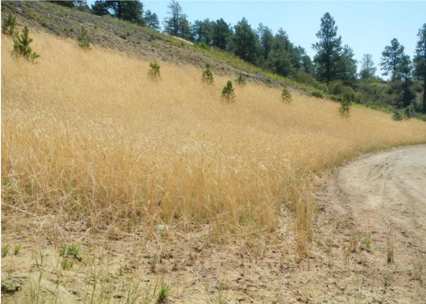
Photo 5. View of cover-crop on lower portion of cut-slope with scattered ponderosa pines ( Pinus ponderosa ). Erosion blankets can be seen in the background and appear to be in disrepair.
