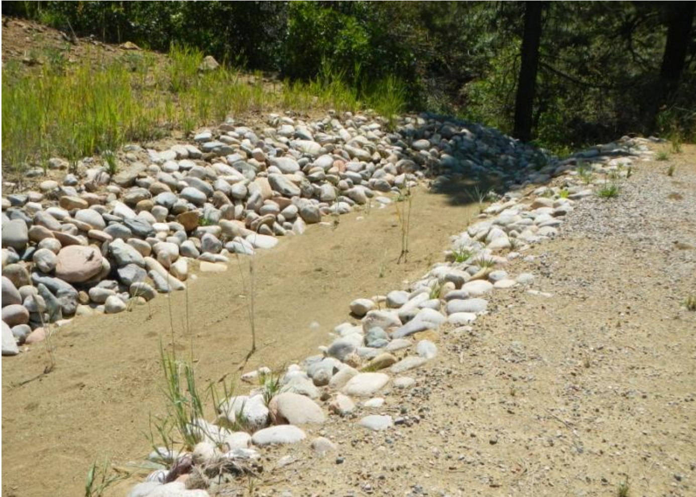
Photo 4. View of Sediment within cut-slope diversion where it flows off of the southern edge of the project area. It appears that sediment is being carried off of the project area.
