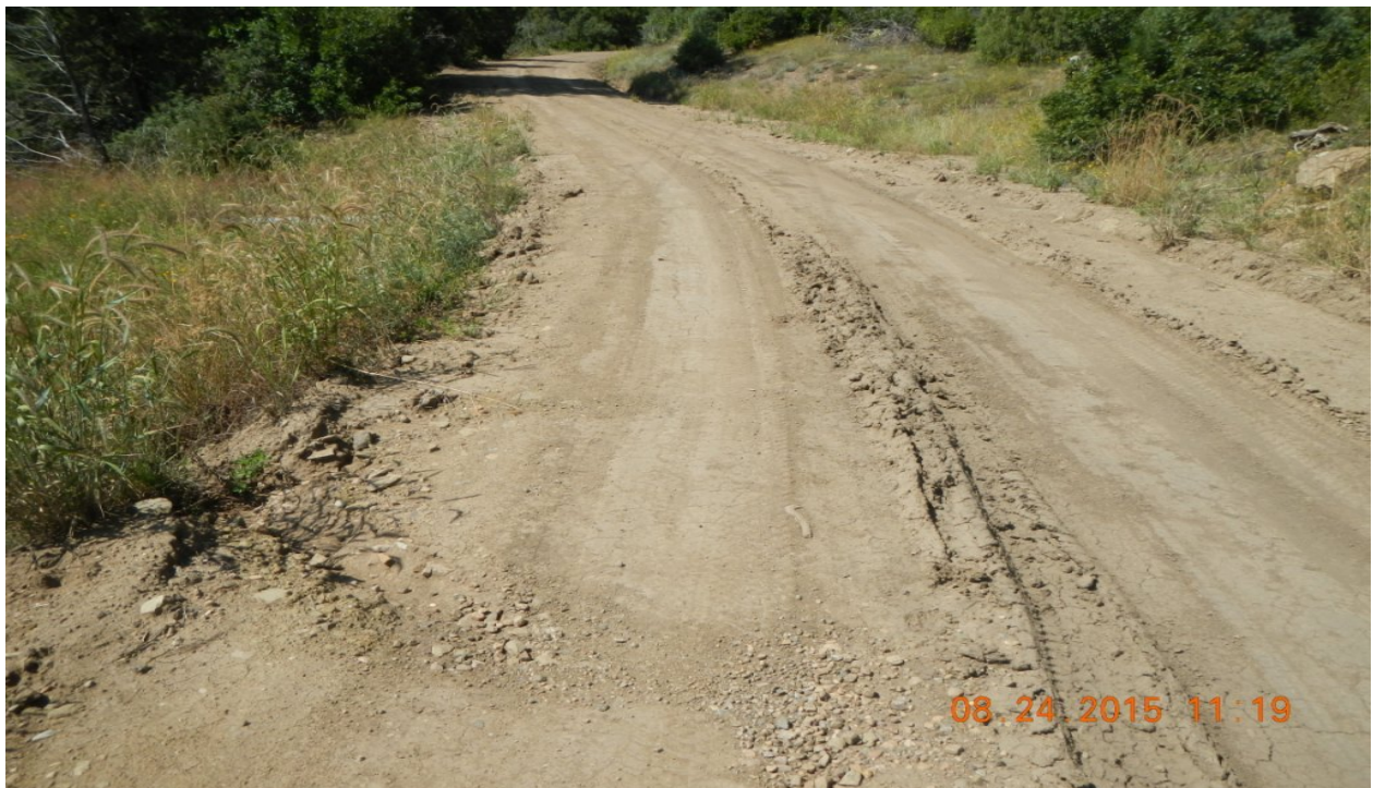
photo 4: Main access road shows signs of erosion and rutting.
