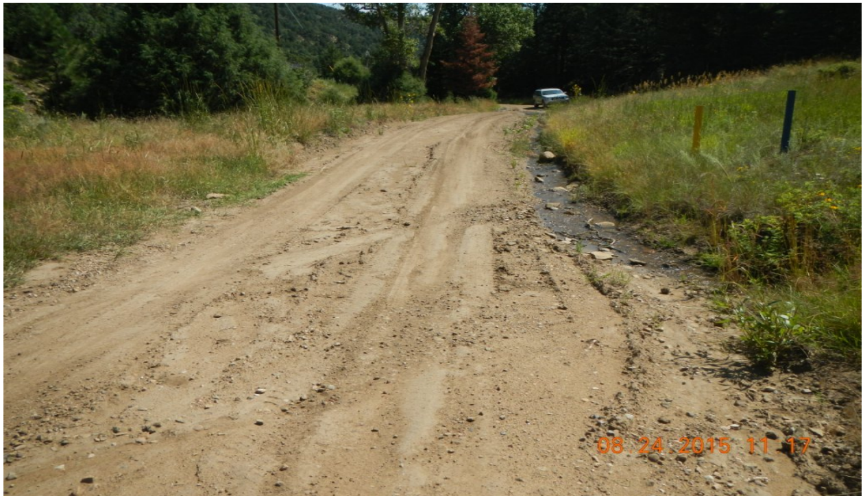
photo 3: There may be a plugged culvert where water source is coming from.
