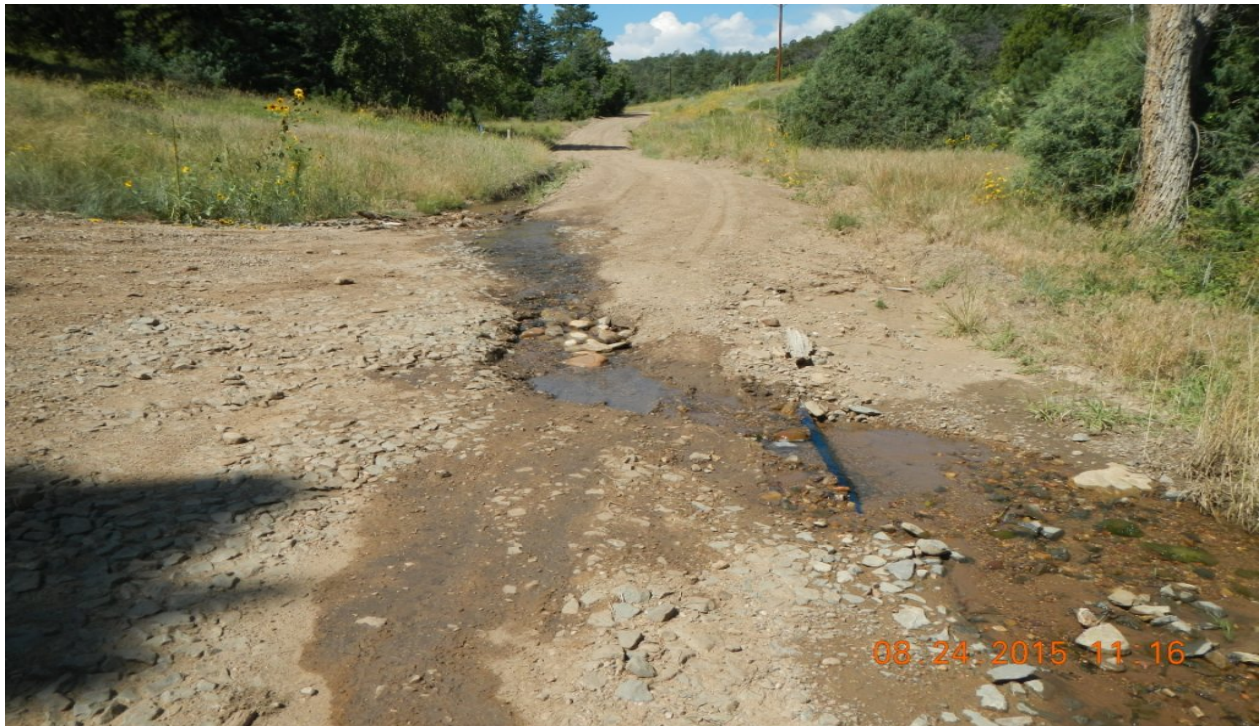
photo 1: Main access road traveling west towards the location. Water is flowing across and eroding the road.
