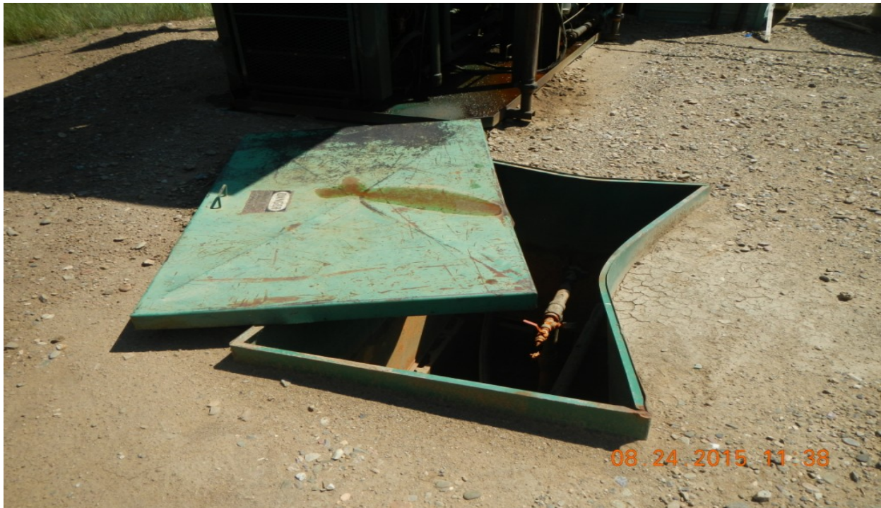
Photo 9: The lid on this cellar near the engine compressor was open and appears to be damaged..
