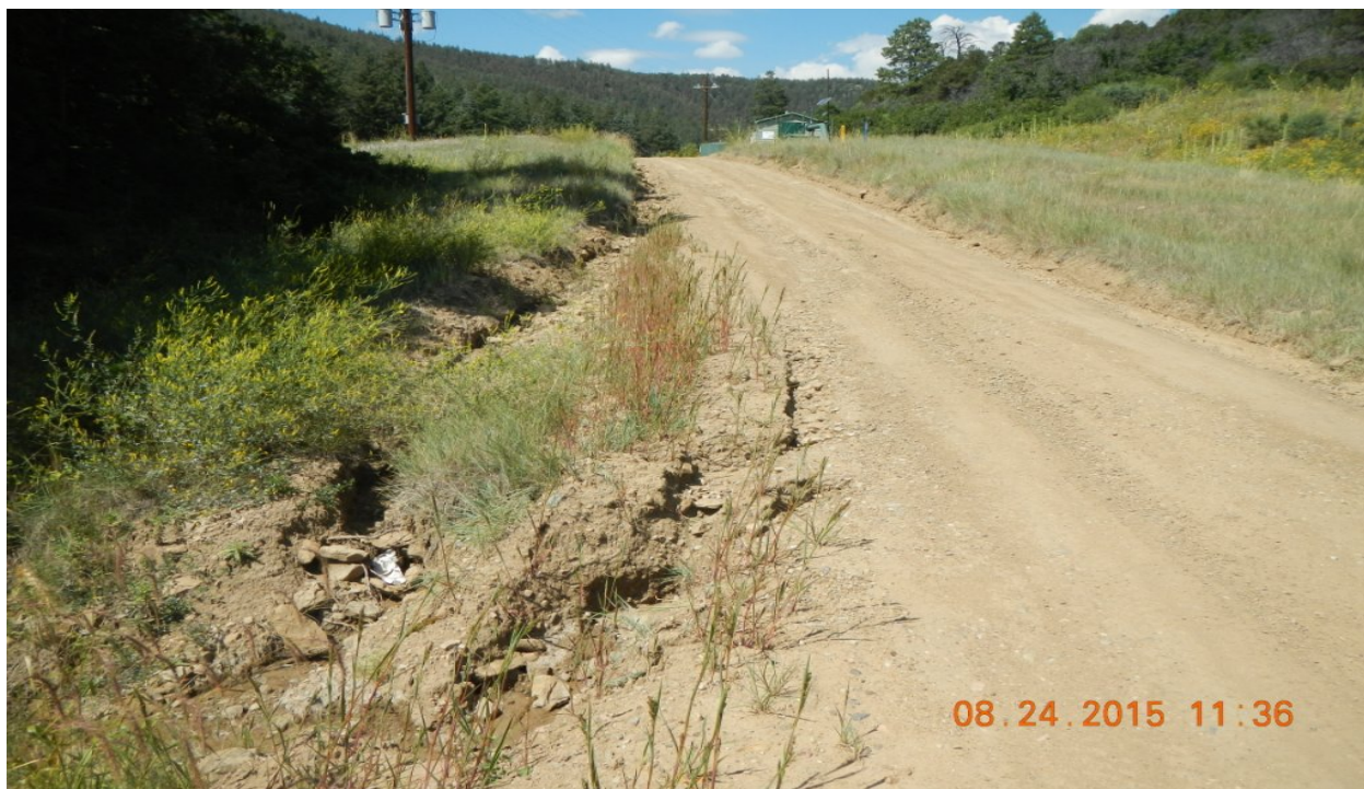
photo 7: Facing west near the location. The main access road shows signs of erosion and vehicle rutting.
