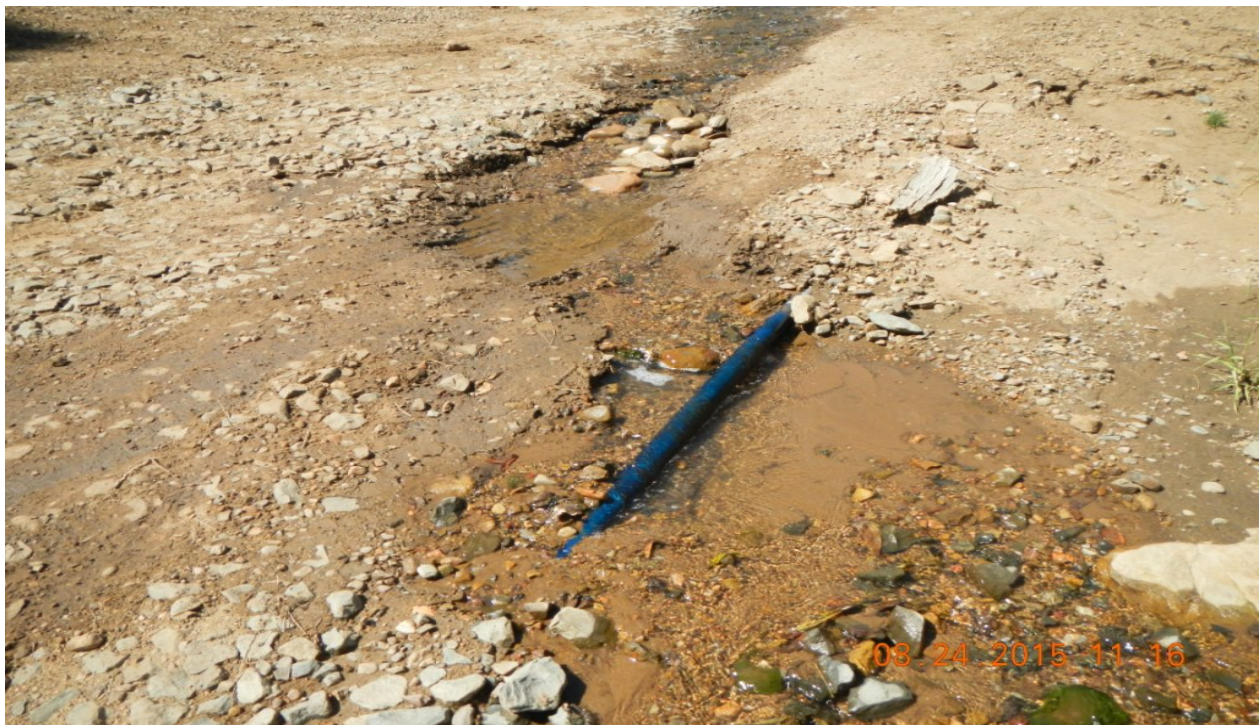
photo 2: Water flowing across the road has exposed a pipeline. Approx. Lat/Long: 37.09117, -104.94348.
